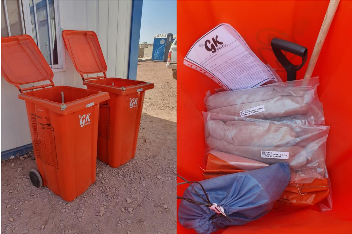
Figure 11: Hydrocarbon Spill Kits must be in place within the site camp and in the field within 500 m of any drilling or ramming activity.
