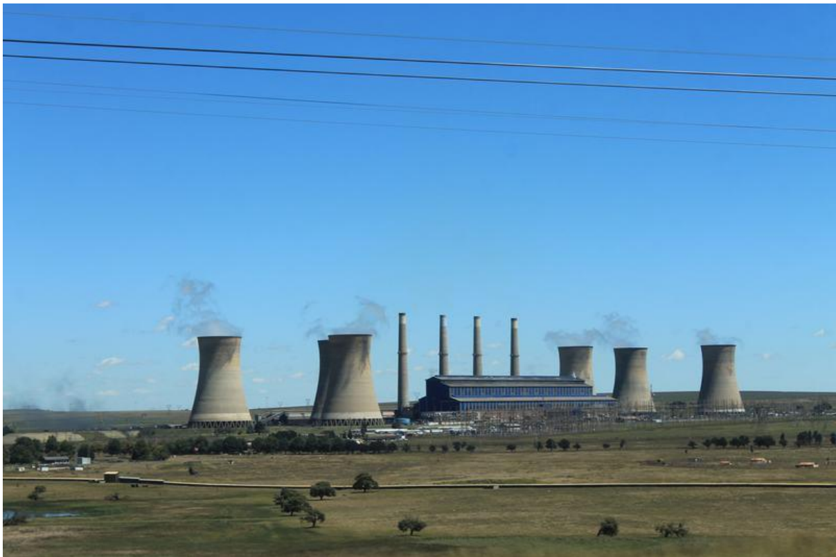
Figure 7-33: Camden Power Station
