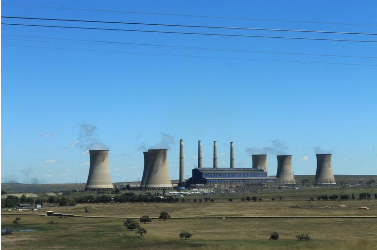
Figure 7.40: Camden Power Station
