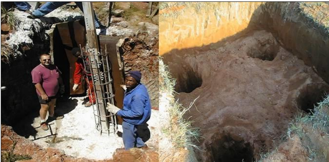
Figure 6.5: Construction of structure foundations
