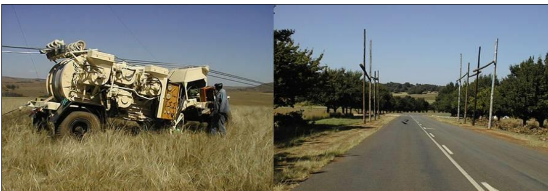
Figure 6.6: Stringing of conductors (power lines)
