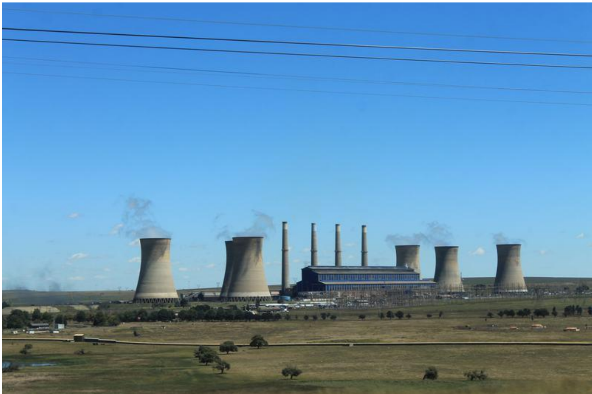
Figure 7.52: Camden Power Station
