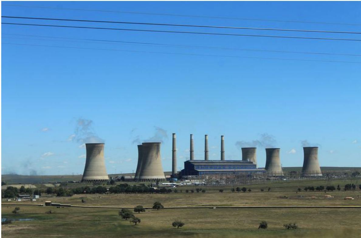
Figure 7-30: Camden Power Station
