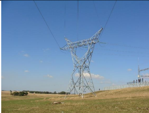
Plate 7-3: Freestanding metal lattice towers.
