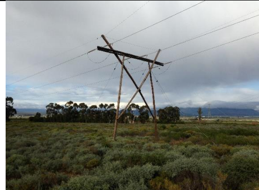
Plate 7-4: Multi-pole structures such as H-towers or K-towers.
