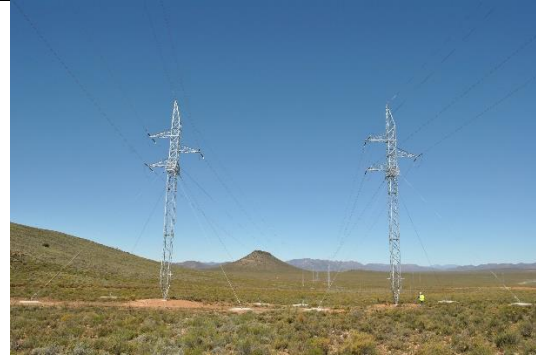
Plate 7-2: Guy line supported steel structures.
