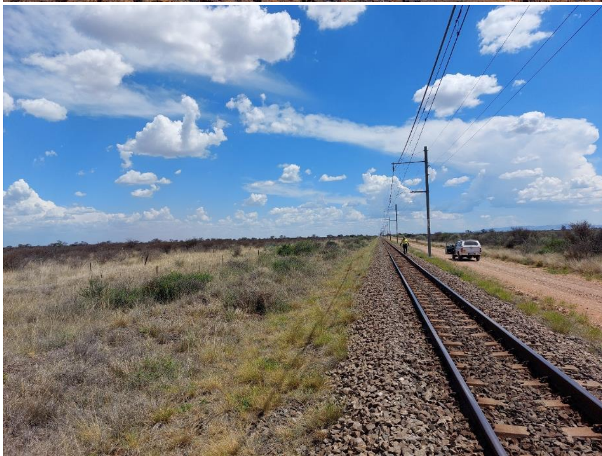
Photograph 1: Infrastructure and vegetation observed on site during the site visit
