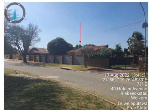
Figure 15: Photo Position 7 situated towards the southwest of the site
