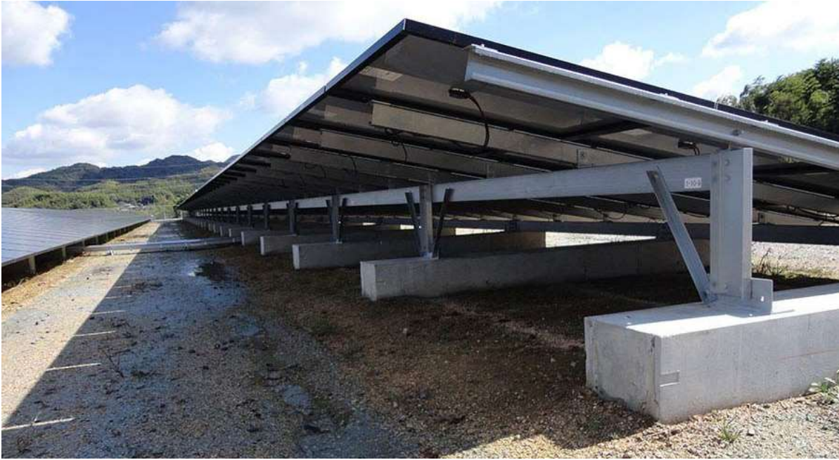
Figure 2: Cast Concrete Foundation - alternative mounting (Euphorbia PV, 2022)
