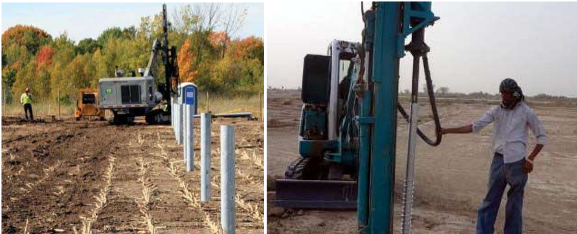
Figure 3: Driven/ Rammed Steel Pile (left) and Ground Screw (right) are the preferred mounting technology (Euphorbia PV, 2022)
