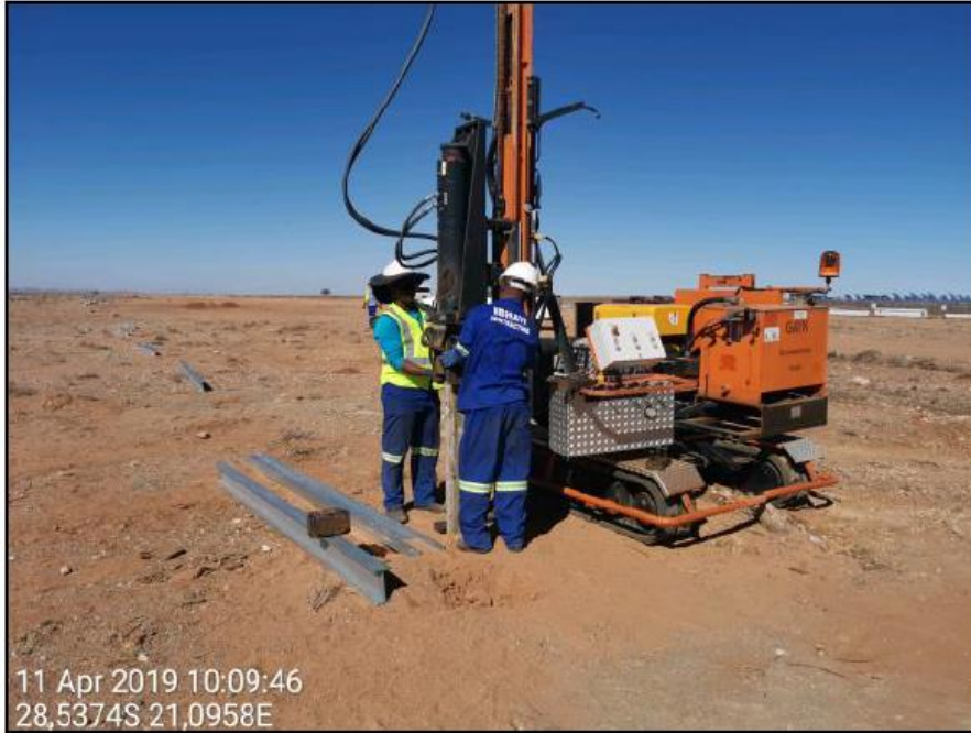
Figure 6: Ramming of steel piles into the pre-drilled / backfilled holes.
