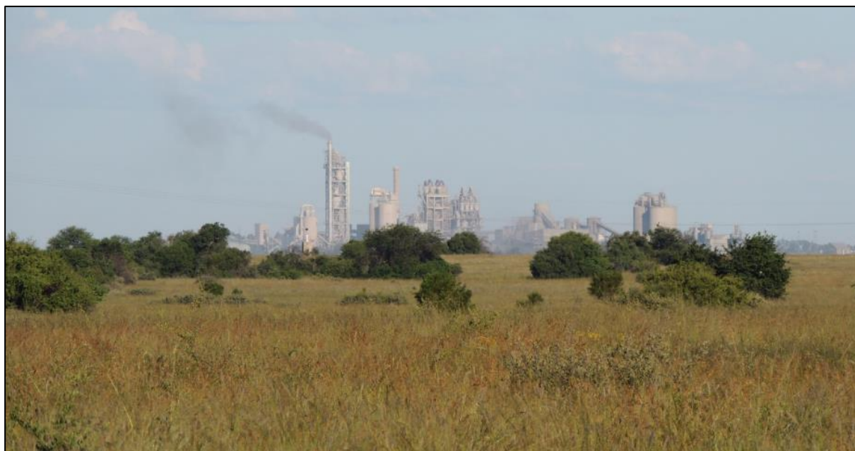
Figure 43. Photograph of the Lichtenburg LaFarge Cement Factory that forms a background view to much of the regional landscape (Stead, 2022)
