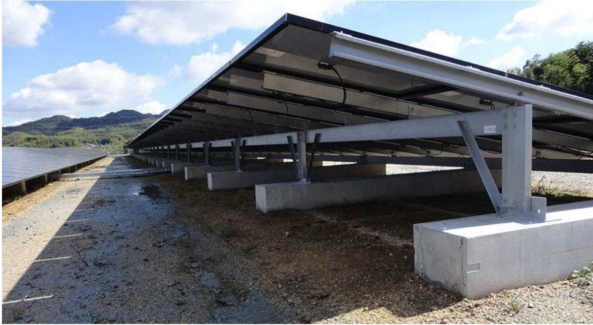
Figure 2: Cast Concrete Foundation - alternative mounting (Hillardia PV, 2022)
