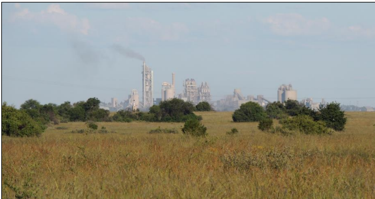
Figure 44. Photograph of the Lichtenburg LaFarge Cement Factory that forms a background view to much of the regional landscape (Stead, 2022)
