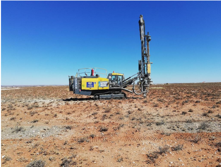
Figure 5: Pre-drilling of holes prior to the ramming of steel piles.
