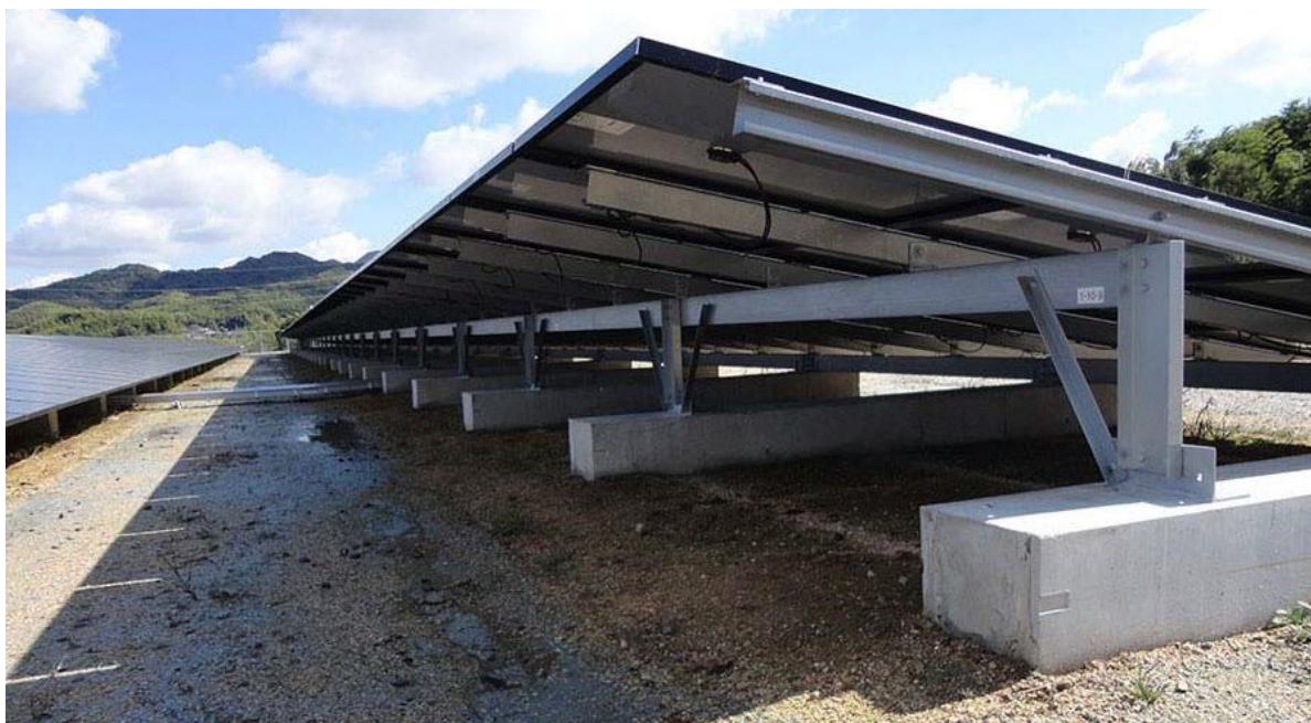
Figure 3: Cast Concrete Foundation - alternative mounting (Verbena PV, 2022)
