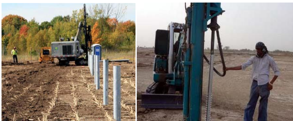
Figure 4: Driven/ Rammed Steel Pile (left) and Ground Screw (right) are the preferred mounting technology (Verbena PV, 2022)
