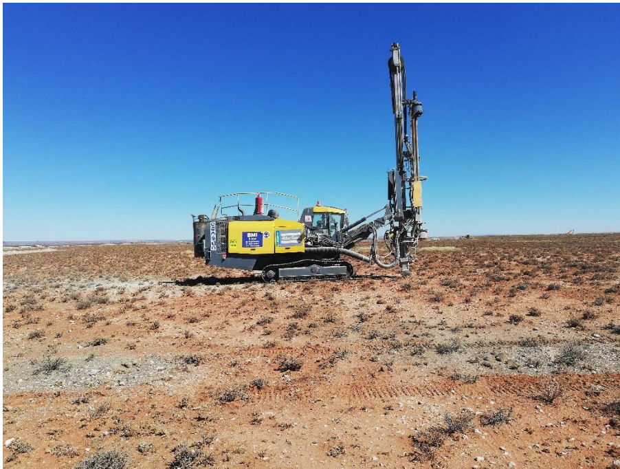
Figure 4: Pre-drilling of holes prior to the ramming of steel piles.
