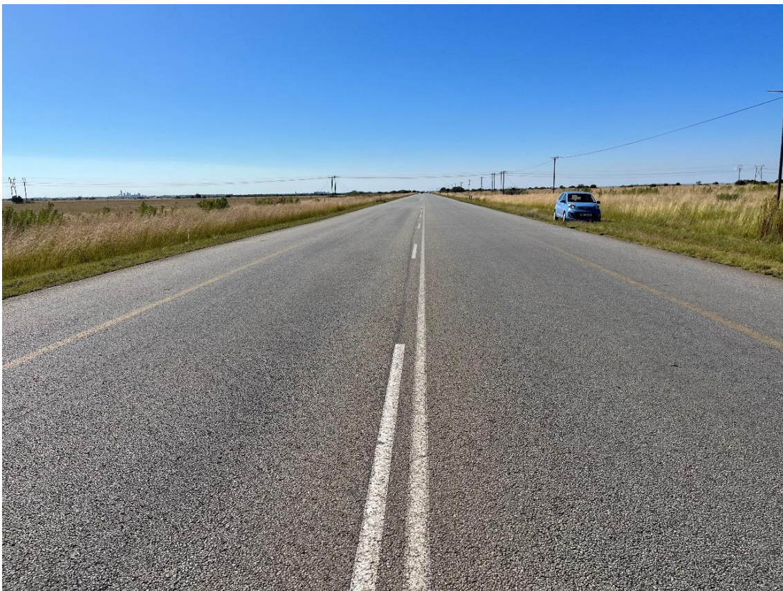
Figure 10: Existing Road P28-4 @ Km 7.15 – East Approaching (Access 1) (Sivest 2022)
