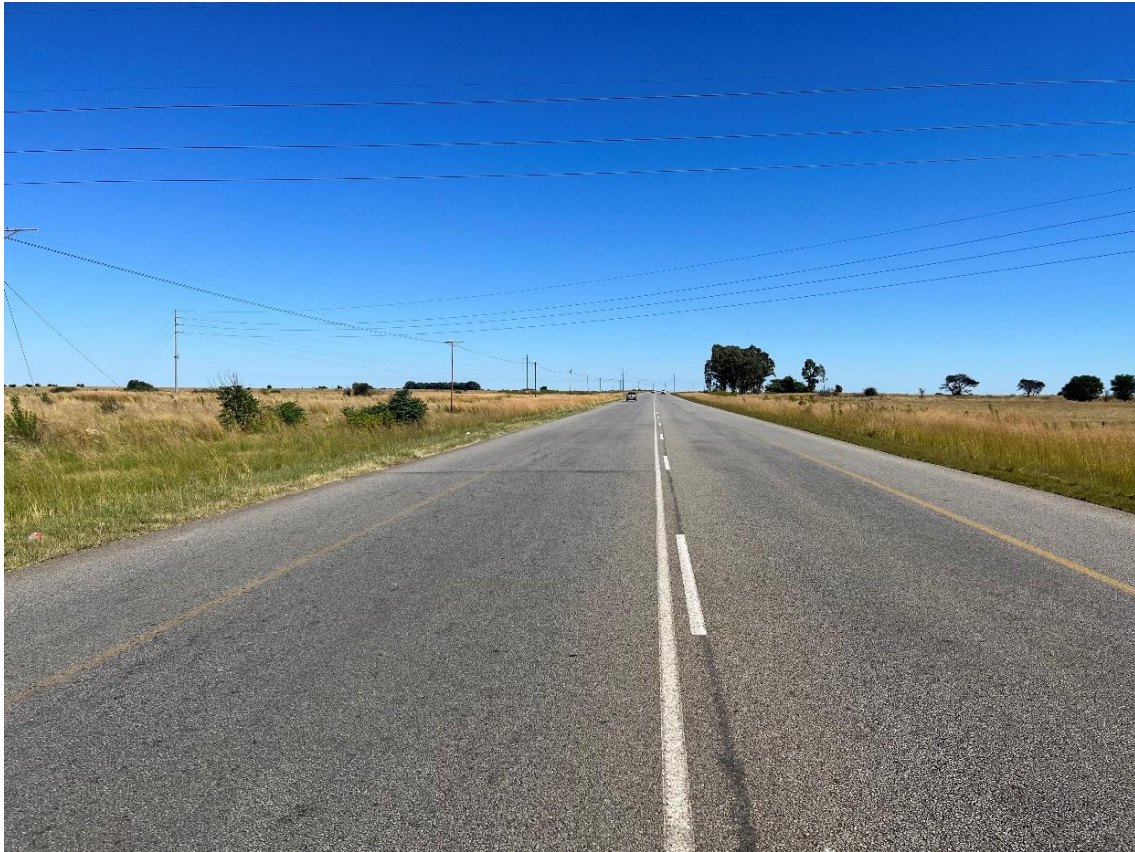
Figure 11: Existing Road P28-4 @ Km 7.15 – West Approaching (Access 1) (SiVEST, 2022)
