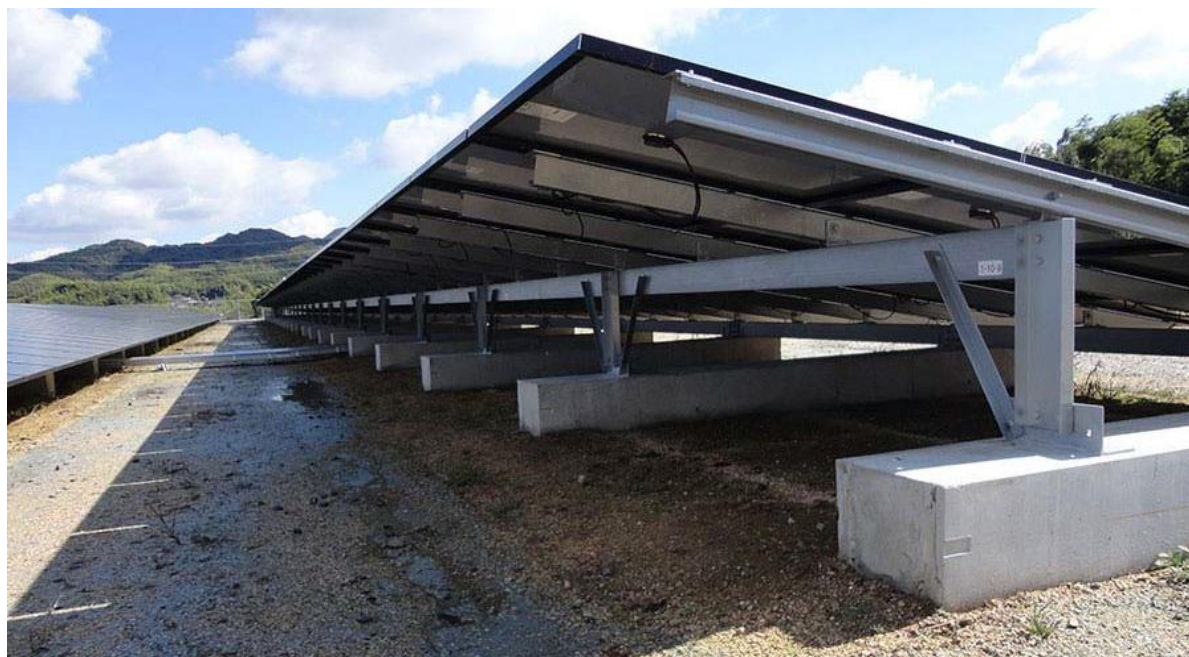
Figure 2: Cast Concrete Foundation - alternative mounting (Themeda PV, 2022)
