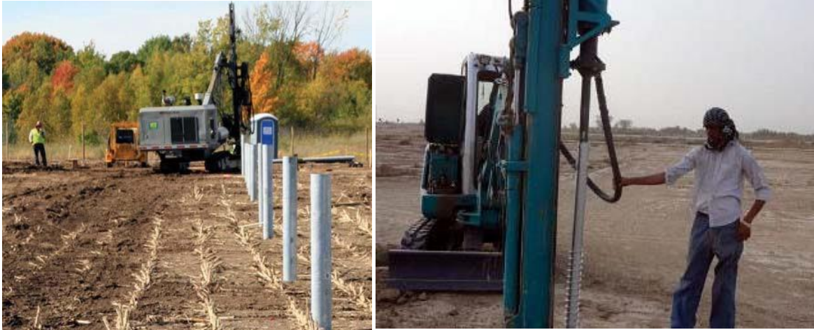
Figure 3: Driven/ Rammed Steel Pile (left) and Ground Screw (right) are the preferred mounting technology (Themeda PV, 2022)
