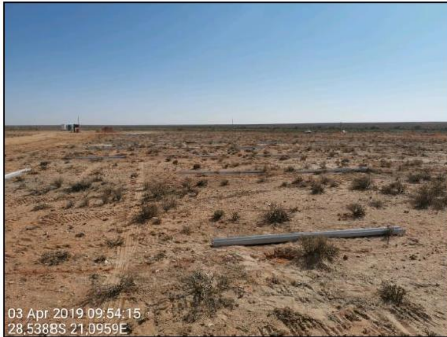
Figure 5: pre-drilled holes are backfilled with a wet sand mixture and steel piles placed in position ready for ramming.
