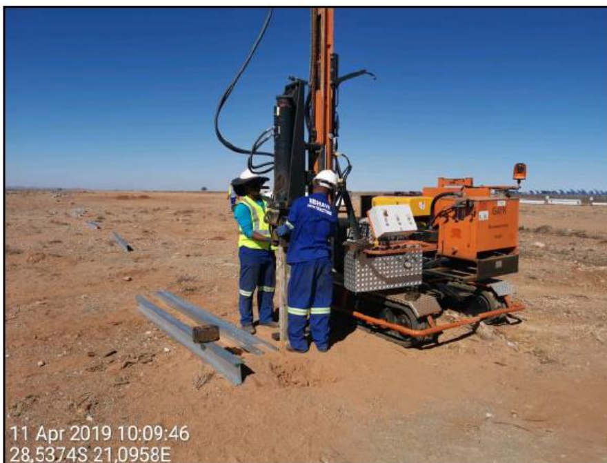
Figure 6: Ramming of steel piles into the pre-drilled / backfilled holes.
