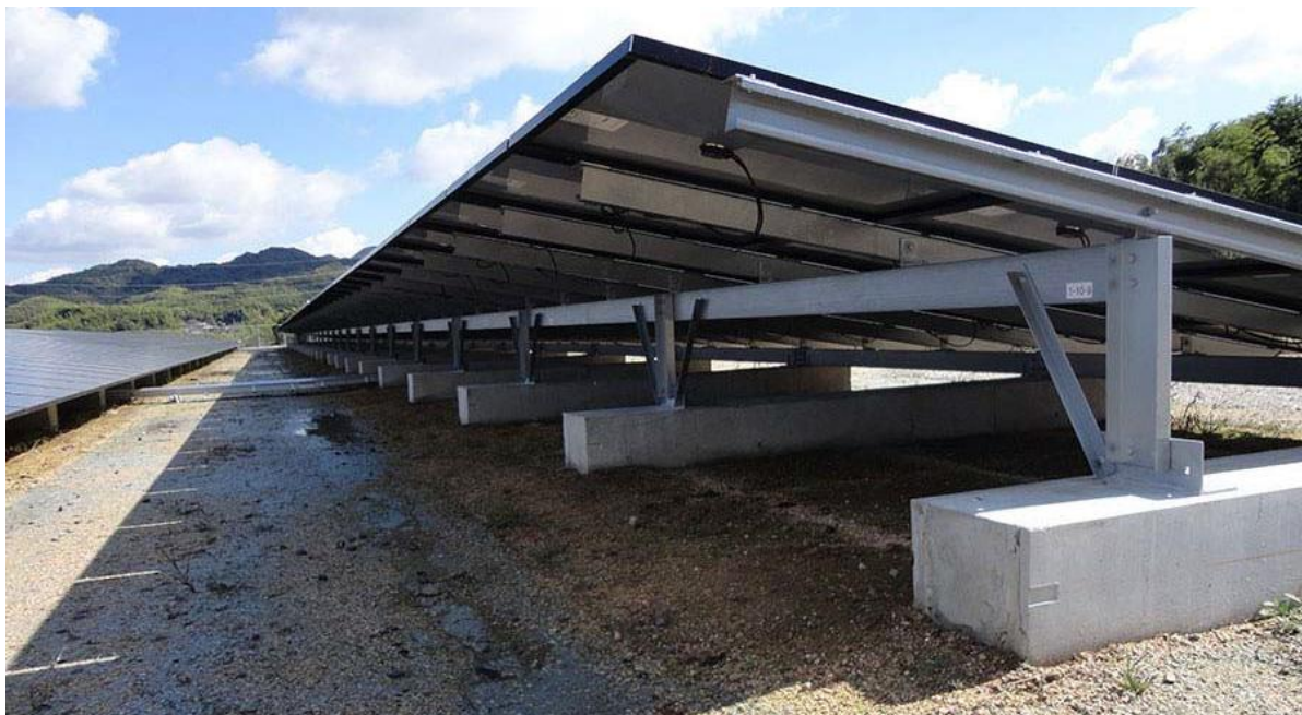
Figure 2: Cast Concrete Foundation - alternative mounting (Themeda PV, 2022)
