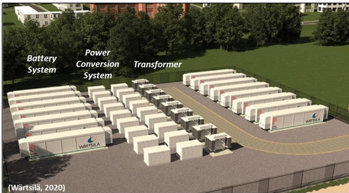
Figure 14: Pivot Power's proposed 50MW lithium-ion battery in Kemsley, Kent.
