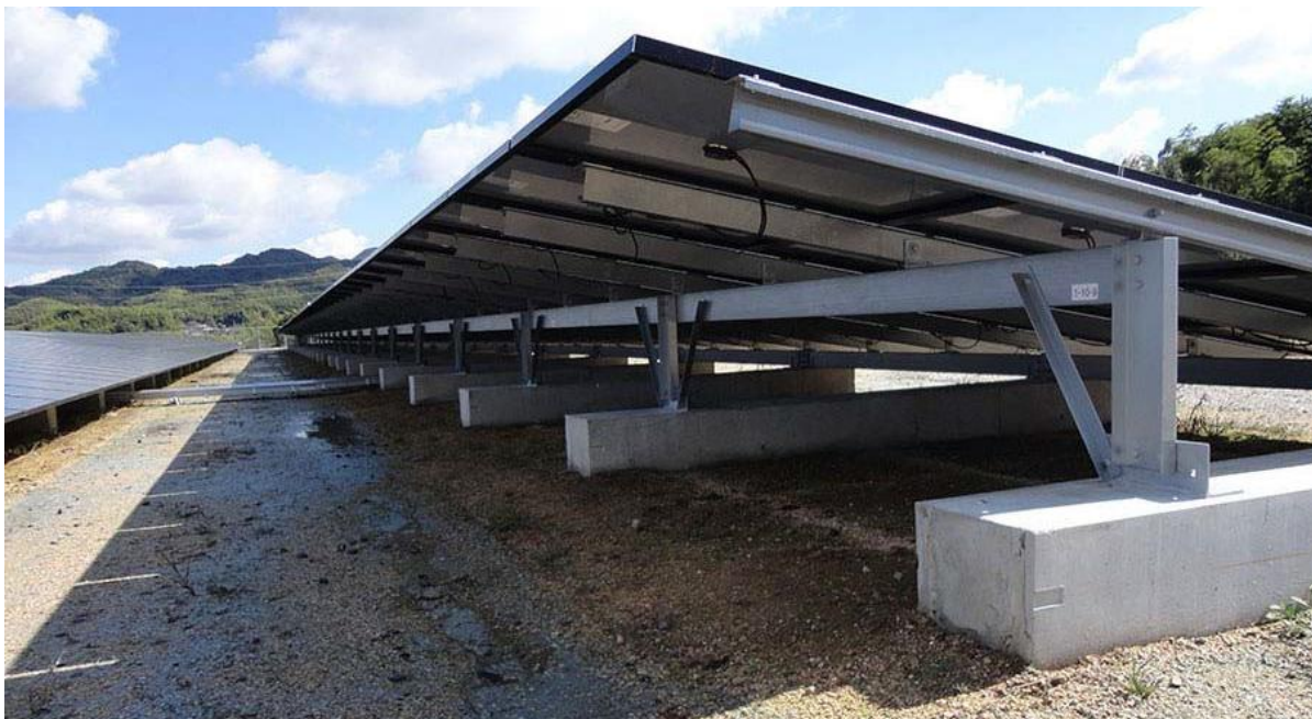
Figure 2: Cast Concrete Foundation - alternative mounting (Aristida PV, 2022)
