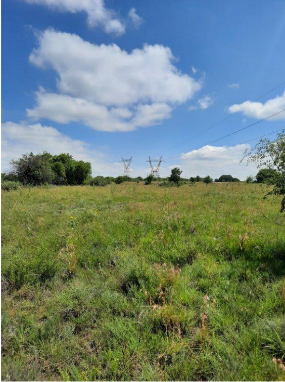
Figure 34: Existing powerlines traversing the Aristida PV site.(van der Walt, 2022).
