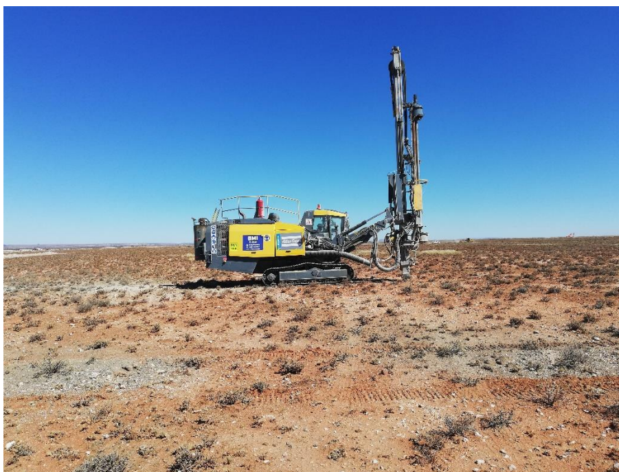
Figure 4: Pre-drilling of holes prior to the ramming of steel piles.
