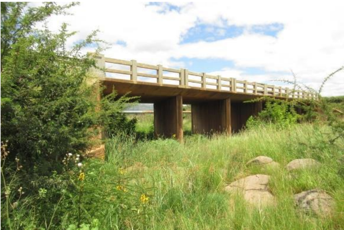
Picture 5: Rooisloot River bridge (7.3.2)
