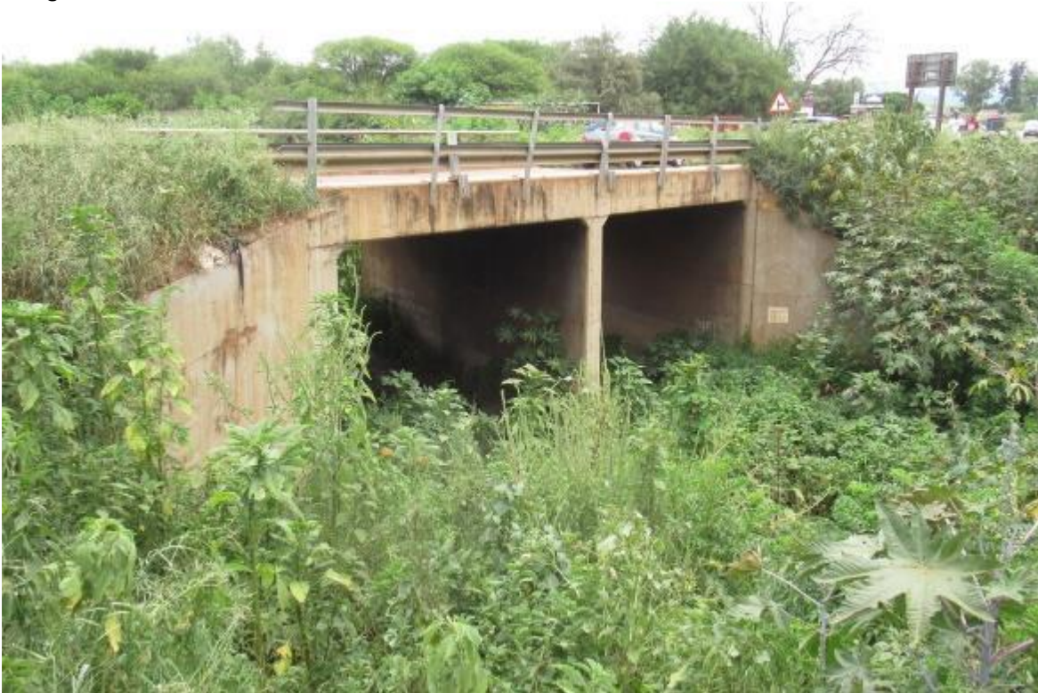
Picture 4: Dorps River bridge (7.3.1)
