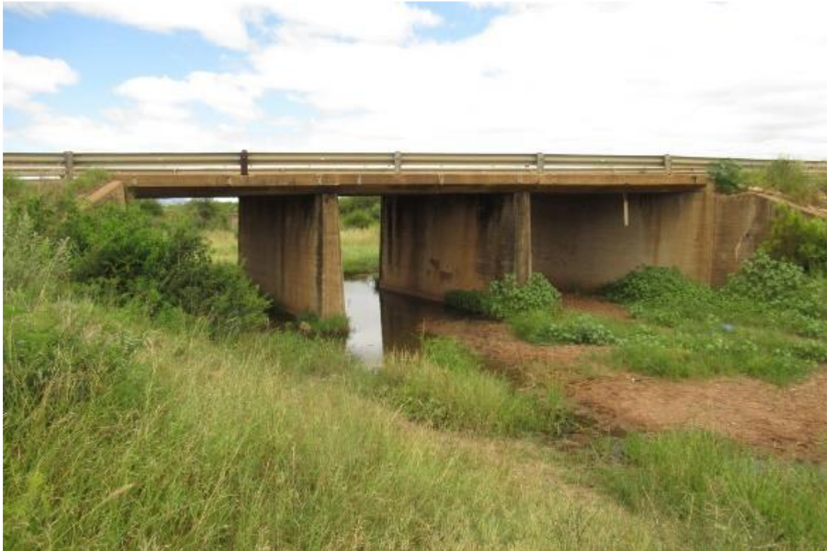
Picture 6: Dithokeng River bridge (7.3.3)
