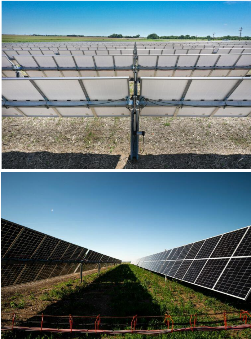
Figure 26: Monofacial (top) and bifacial (bottom) solar panels ( https://www.bluestemenergysolutions.com/bifacial-versus-monofacial-solar-panels-an-analysis/ )
