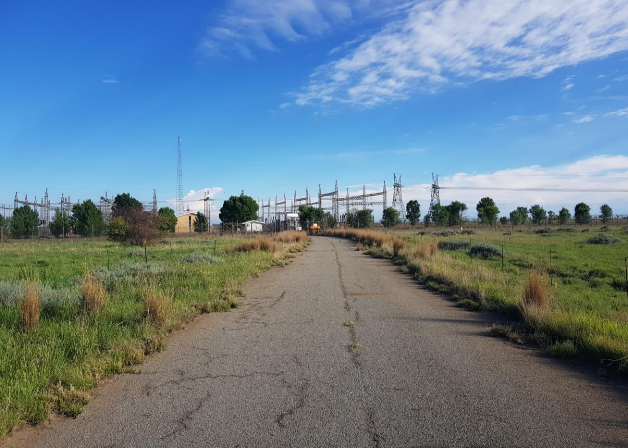
Figure 45: Existing Eskom Substation
