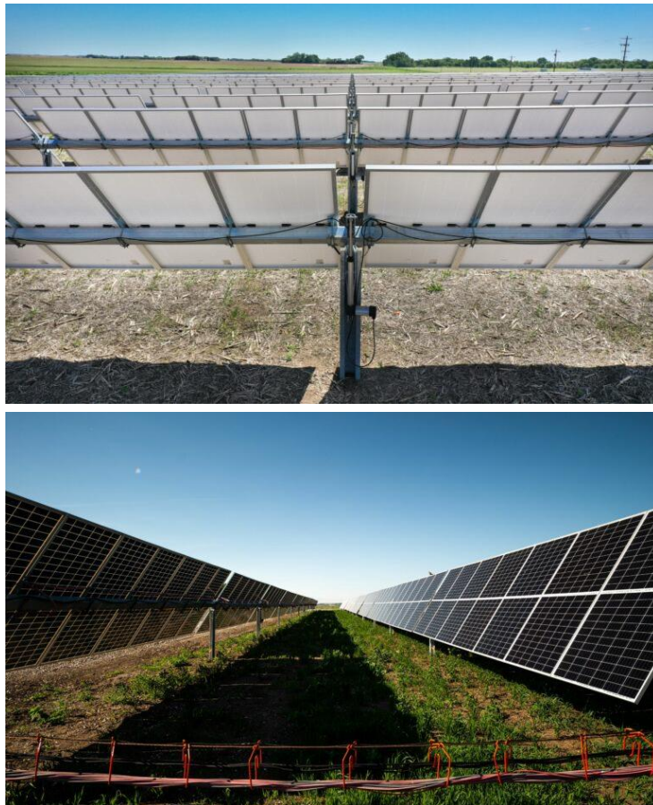
Figure 20: Monofacial (top) and bifacial (bottom) solar panels
