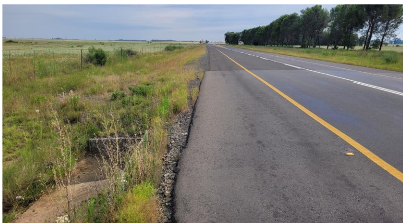
Figure 52: Northern view along the N6 (PV Site on left-hand side)
