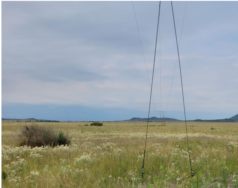
Figure 51: Western view of the PV Site showing existing power line
