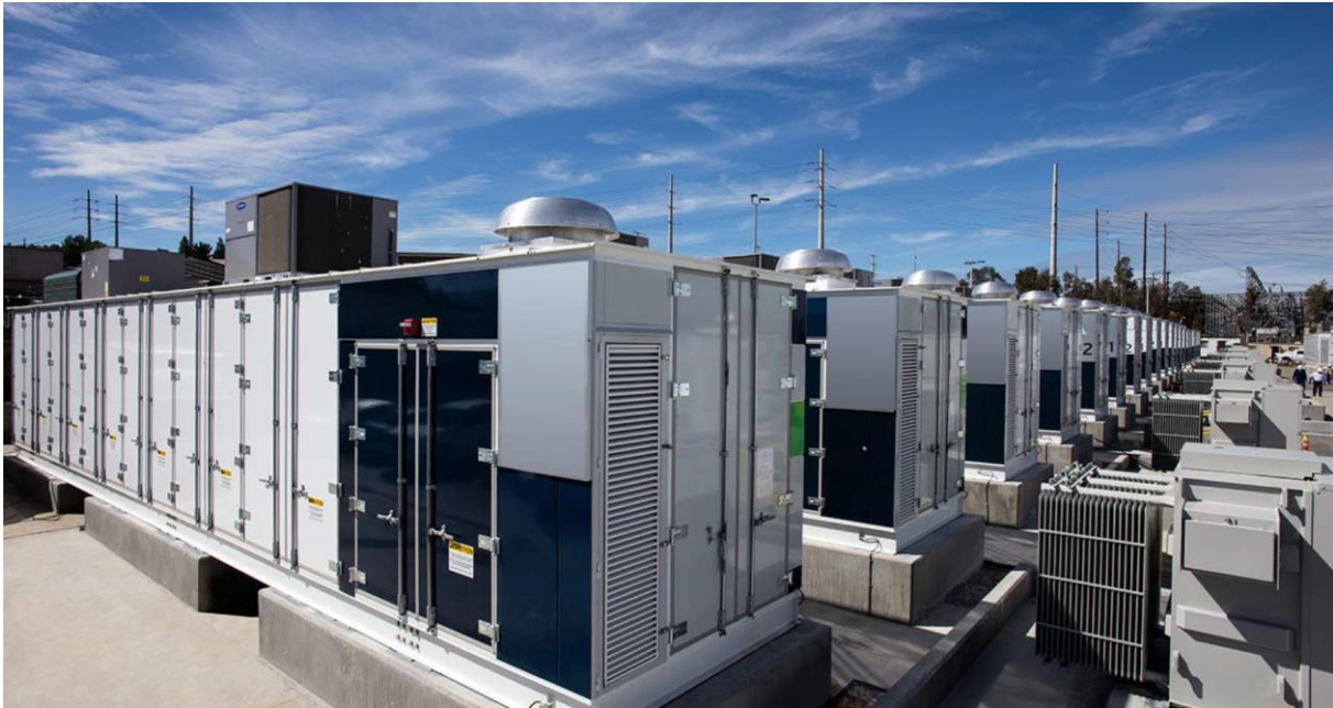
Figure 16: Example of BESS installation ( https://biiworld.com/ )
