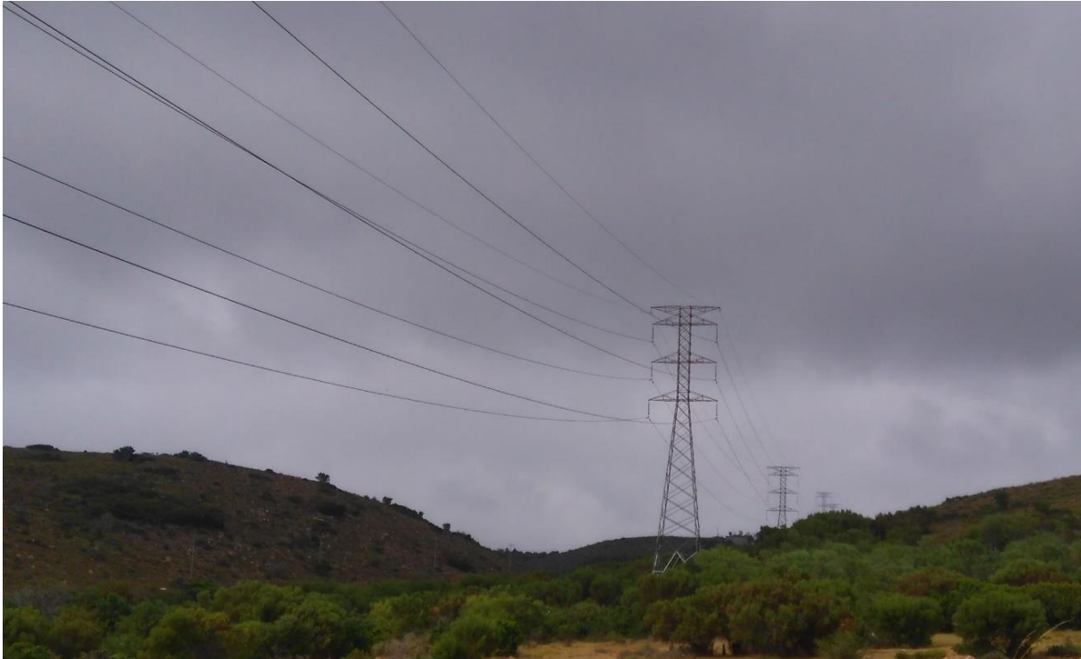
Figure 17: Example of a 132 kV transmission line
