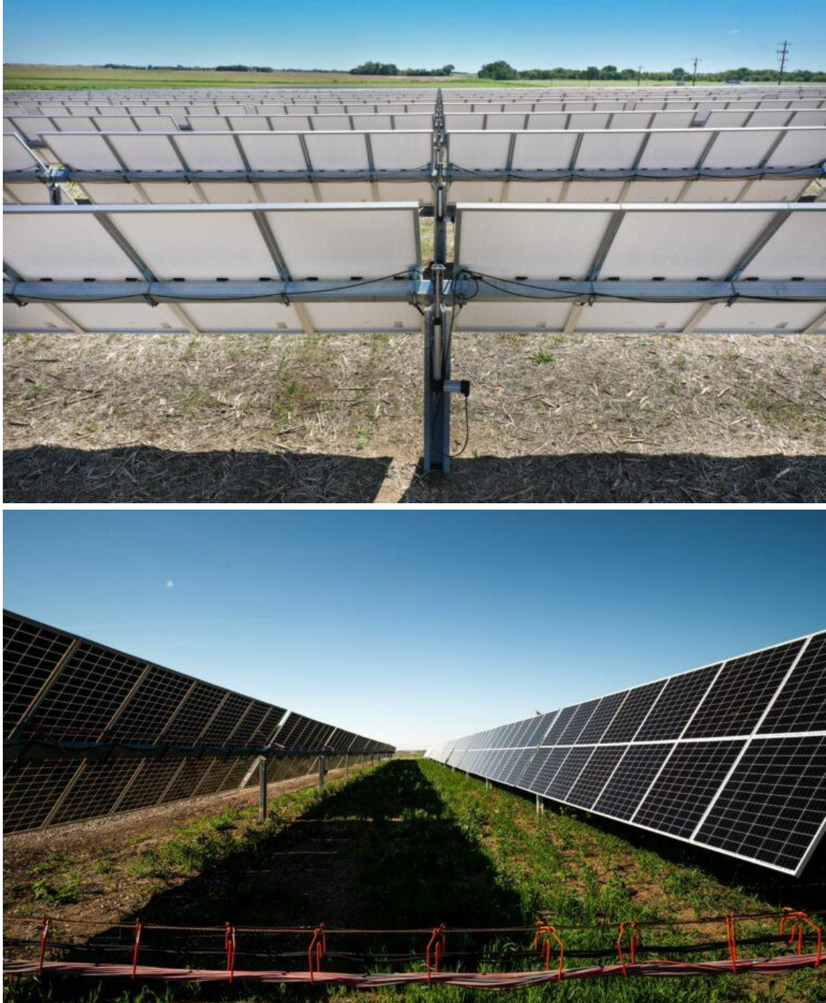
Figure 20: Monofacial (top) and bifacial (bottom) solar panels
