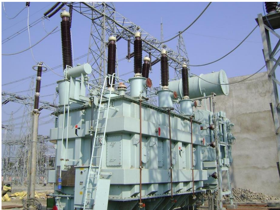
Figure 11: Example of Medium Voltage Transformer (source: https://www.ulaginoli.com/ )
