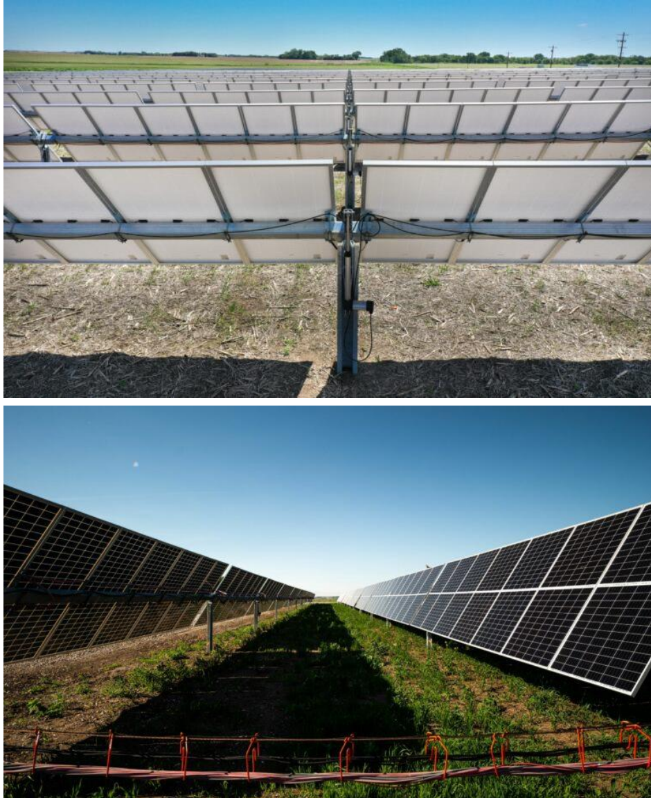
Figure 21: Monofacial (top) and bifacial (bottom) solar panels
