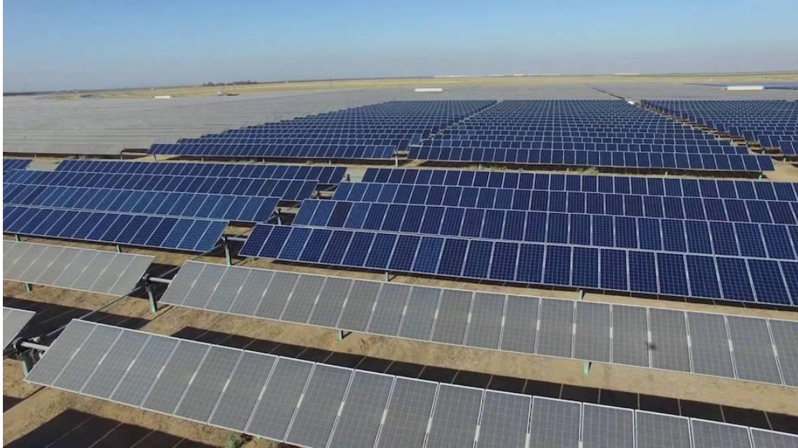
Figure 14: Example of Roads Between Trackers and Medium Voltage Substations (source: https://ecoinventos.com/ )
