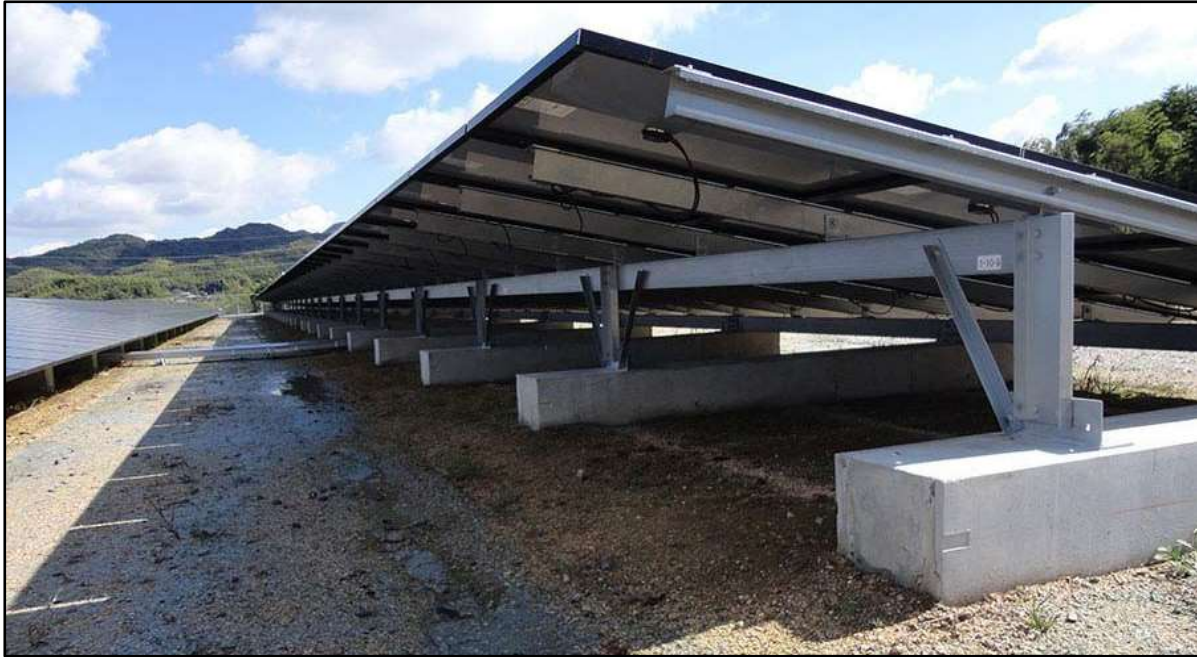
Figure 3: Cast Concrete Foundation (alternative mounting)
