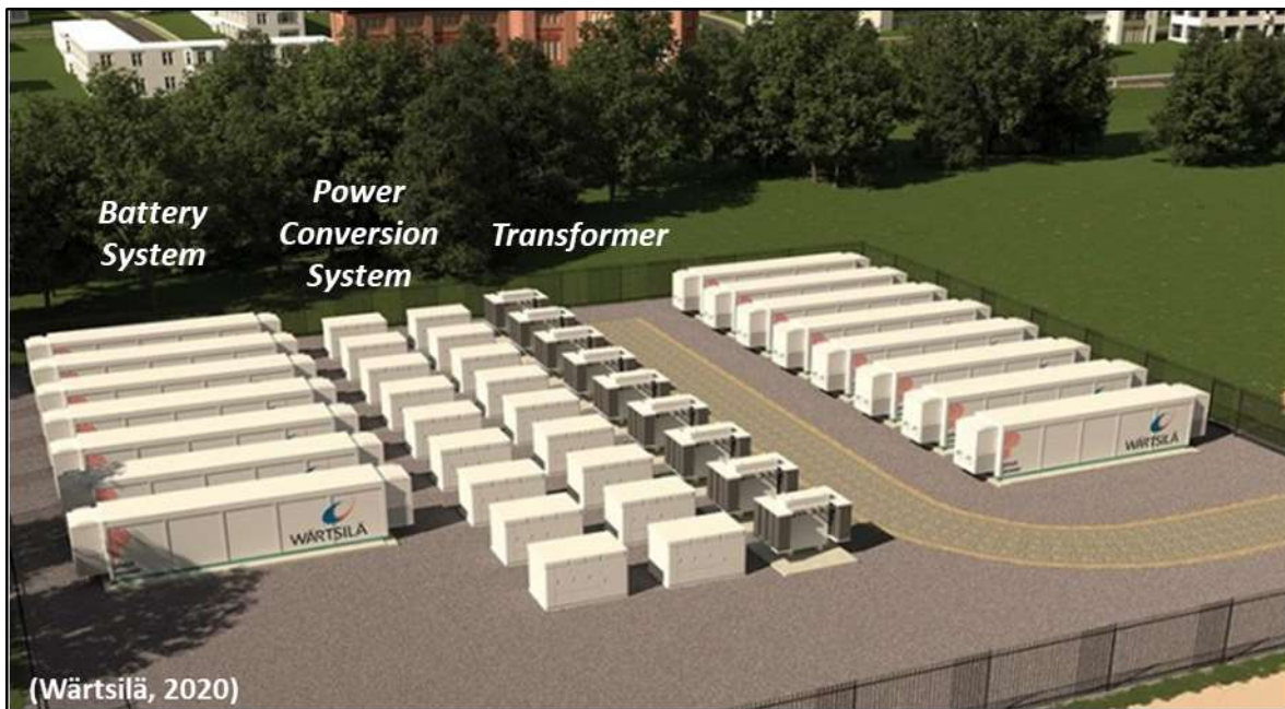
Figure 7: Pivot Power's proposed 50MW lithium-ion battery energy storage system in Kemsley, Kent.
