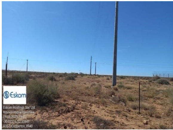
Figure 2-6: Other existing infrastructure near Kronos substation
