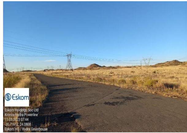
Figure 2-7: Access Road to Hydra substation
