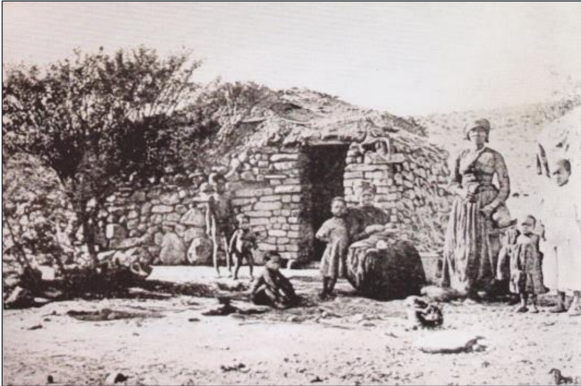
Figure 6-19 - A shepherd's hut photographed near Beaufort West in the early 20th century. Note the low, narrow doorway and informal roof structure. Source: Schoeman (2013:48)
