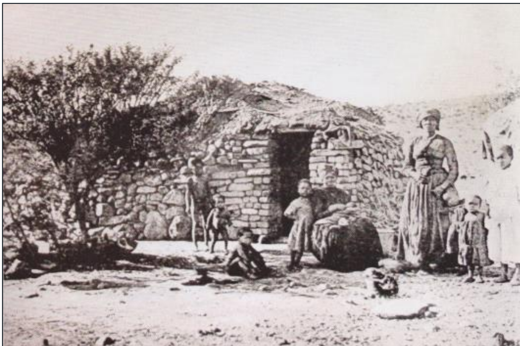
Figure 6-20 - A shepherd's hut photographed near Beaufort West in the early 20th century. Note the low, narrow doorway and informal roof structure. Source: Schoeman (2013:48)
