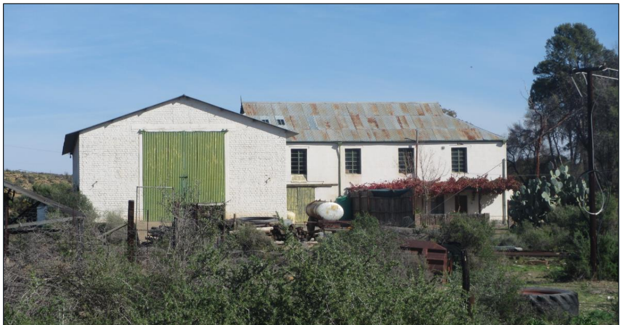
Figure 6-35 - An unusual double story structure in the Boiskraal Farm complex at Waypoint 1794. Source: Orton (2021a: fig. 51)
