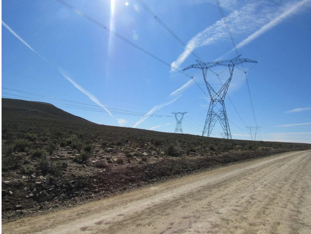
Figure 6-47: View of high voltage power lines in the study area
