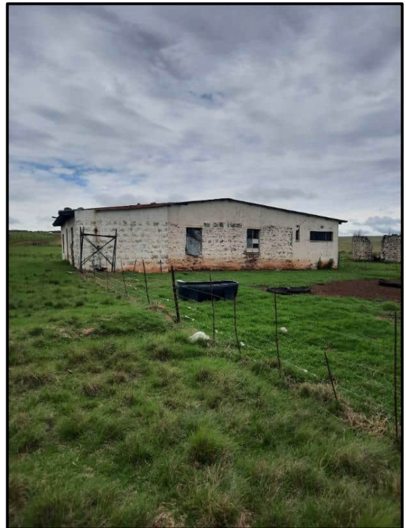
Figure 7.79. Structure at DN073
