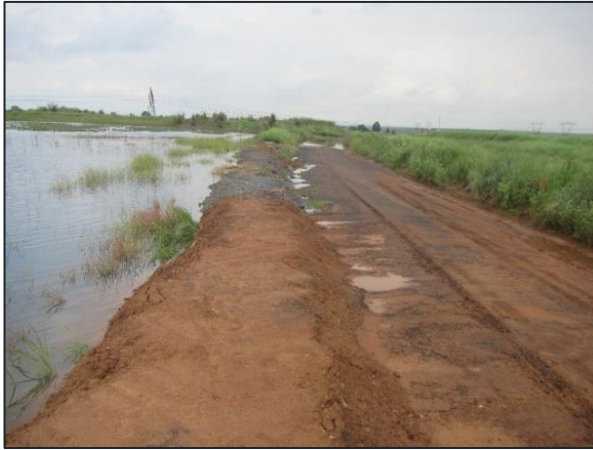
Figure 7-27: Amongst other features, gravel roads and drainage trenches have fragmented habitat in the local study area, and facilitated alien invasive species colonisation
