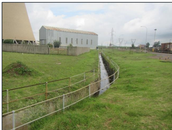
Figure 7-42 - Landscaped lawns adjacent to the Komati cooling towers
