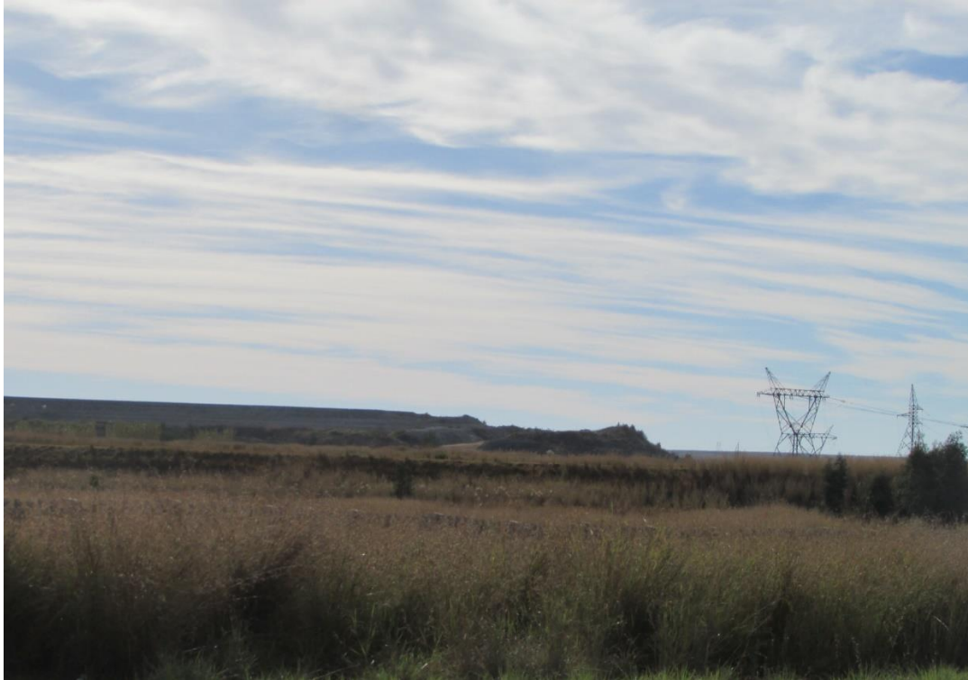
Figure 7-86: A view of the area with the Ash Discard Dump visible (APAC, 2023)
