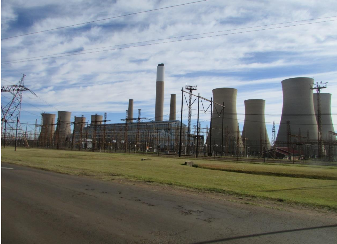
Figure 7-83: A view of the Komati Power Station (APAC, 2023)
