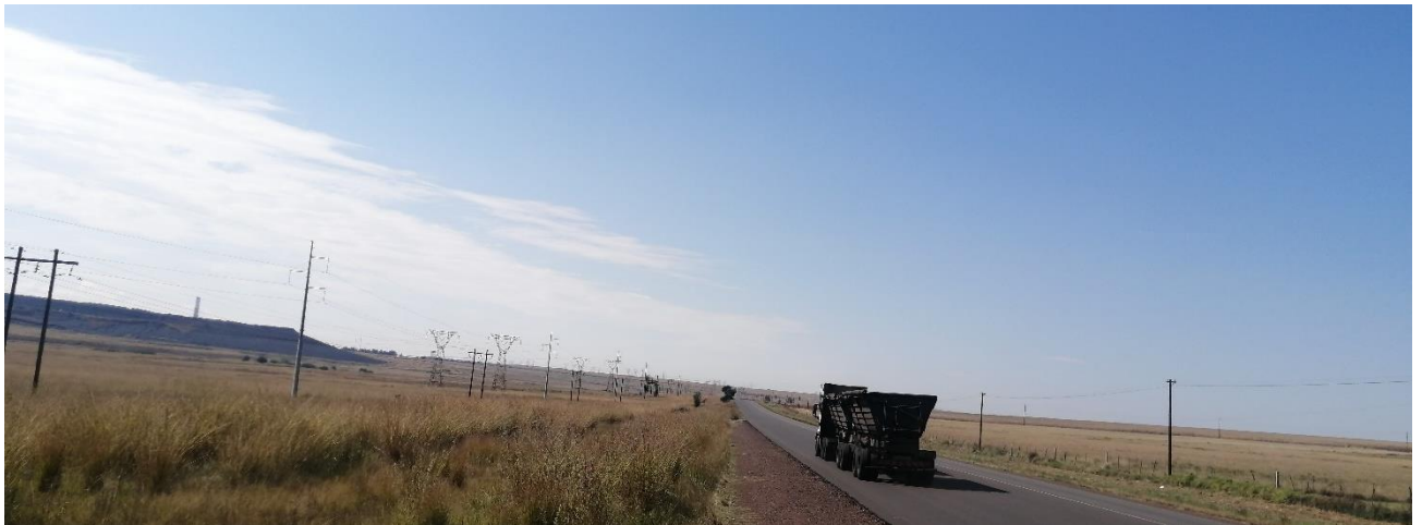
Figure 7-77: View from the R542 towards the site from the west (LOGIS, 2023)
