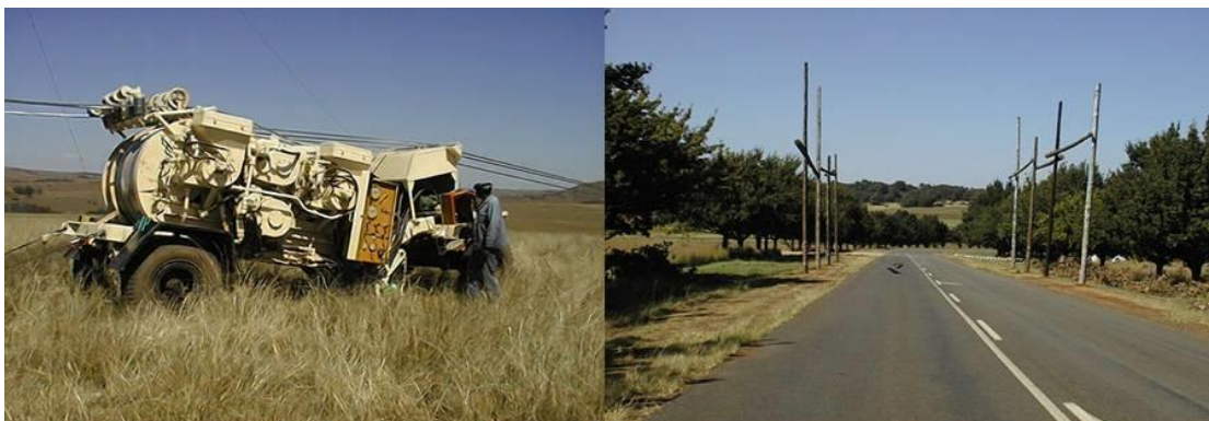
Figure 2-6: Stringing of conductors (power lines)
