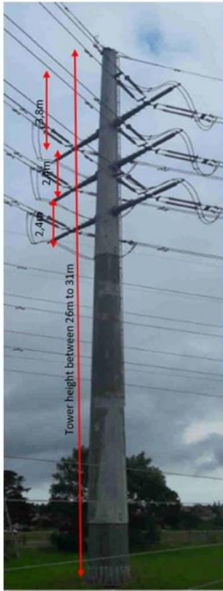
Figure 2-13: In-line or angle-strain self-supporting monopole (double circuit) (illustrative only, subject to detailed design)
