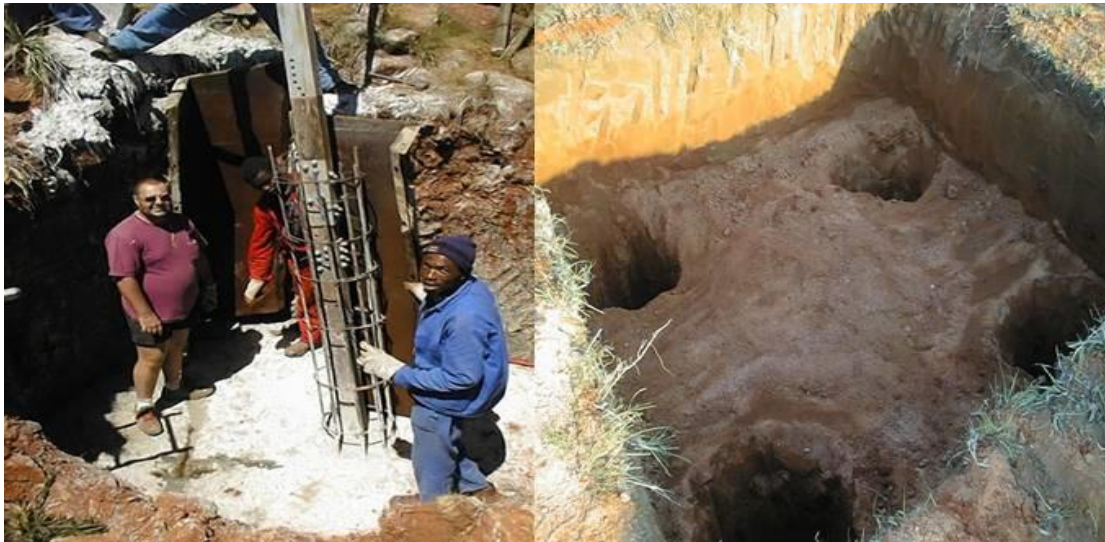
Figure 2-5: Construction of structure foundations
