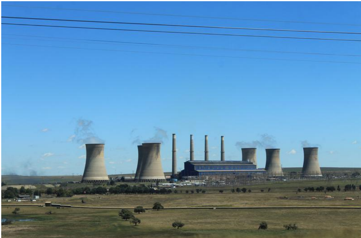
Figure 5-23: Camden Power Station
