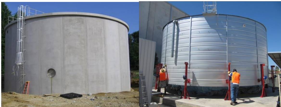
Figure 2-9: Typical water reservoir (left - concrete, right - steel)
