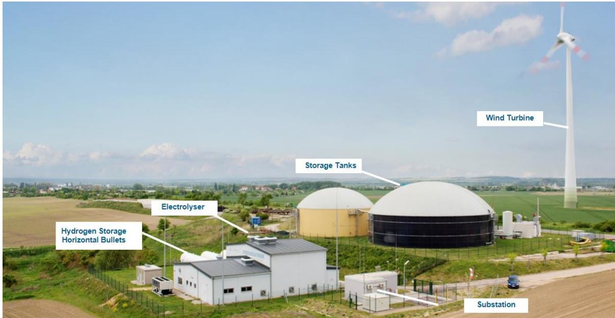
Figure 2-3: Enertrag Germany's Hybridkraftwerk
