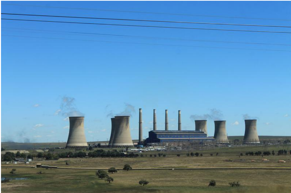
Figure 5-24: Camden Power Station
