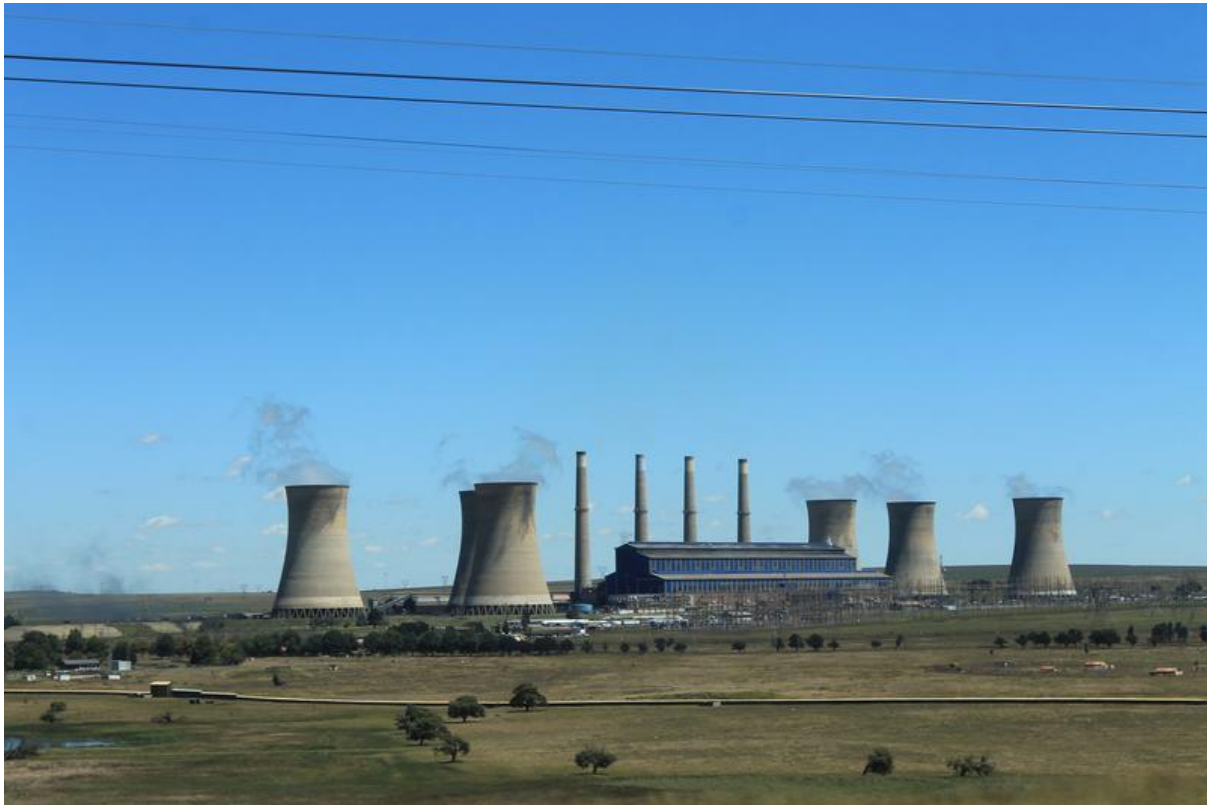
Figure 5-26: Camden Power Station
