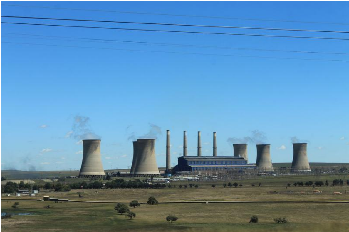
Figure 5-28: Camden Power Station
