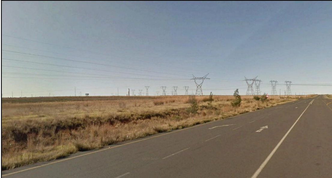
Figure 5.49: Power lines near the R542 arterial road
