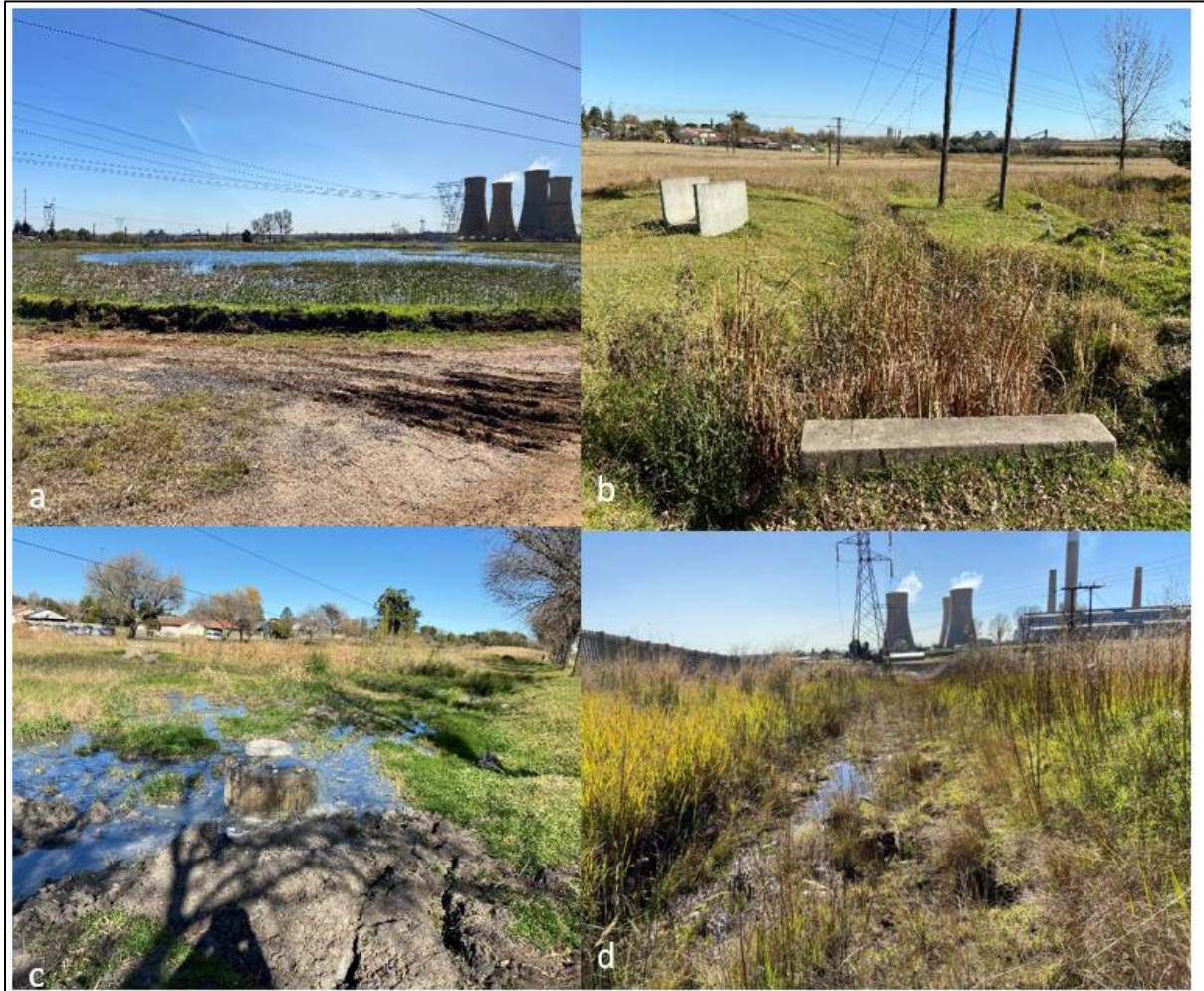
Figure 5.38: Impacts: a) pooling of water at dam; b) trenches and berms in wetland; c) effluent discharge into the wetland from a leaking pipe; d) impoundment of water at roads in wetland
