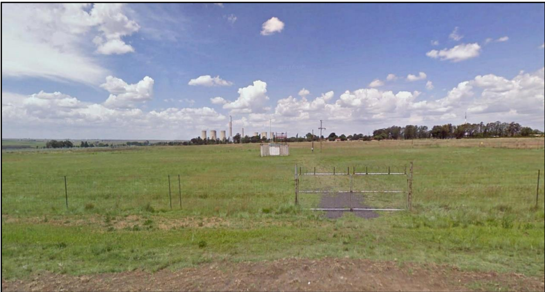
Figure 5.46: View of the PV Site B from the west
