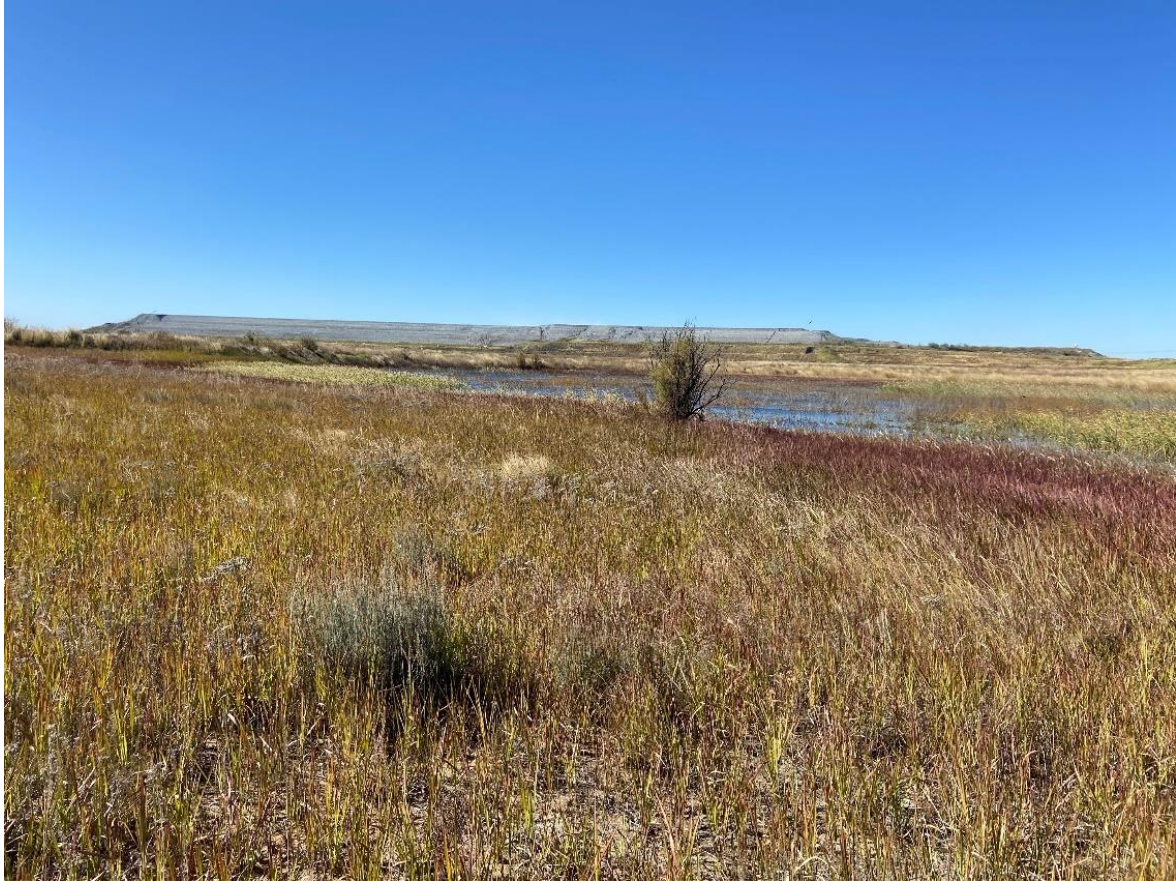
Figure 5.37: Ash dam facility and pooling of water at dam
