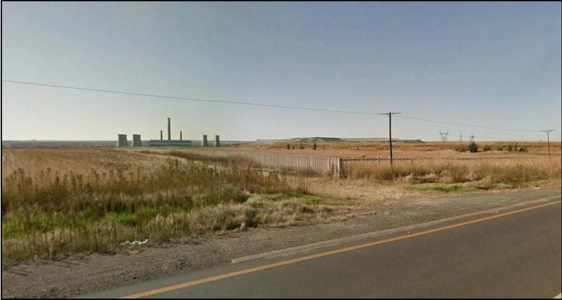
Figure 5.45: View of the PV Site A from the R542 arterial road (LOGIS, 2022)
