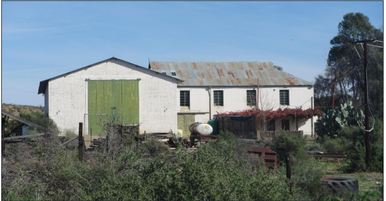
Figure 6-26 - A structure built of stone, sun-dried mud bricks and fired clay bricks at Waypoint 1993
