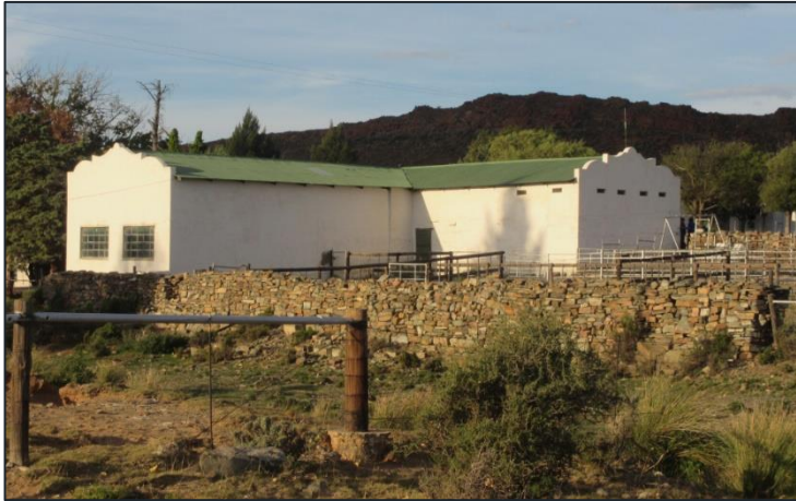
Figure 6-22 - Structure in the Leeukloof Farm complex at Waypoint 1850
