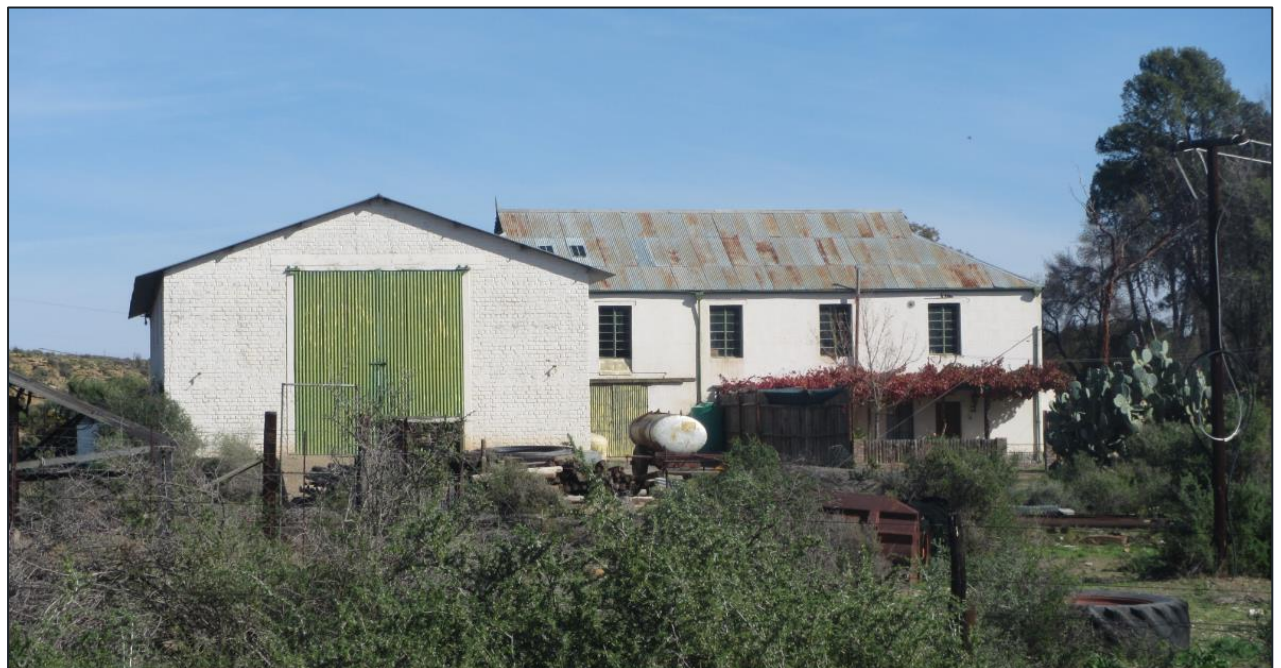
Figure 6-24 - A structure built of stone, sun-dried mud bricks and fired clay bricks at Waypoint 1993
