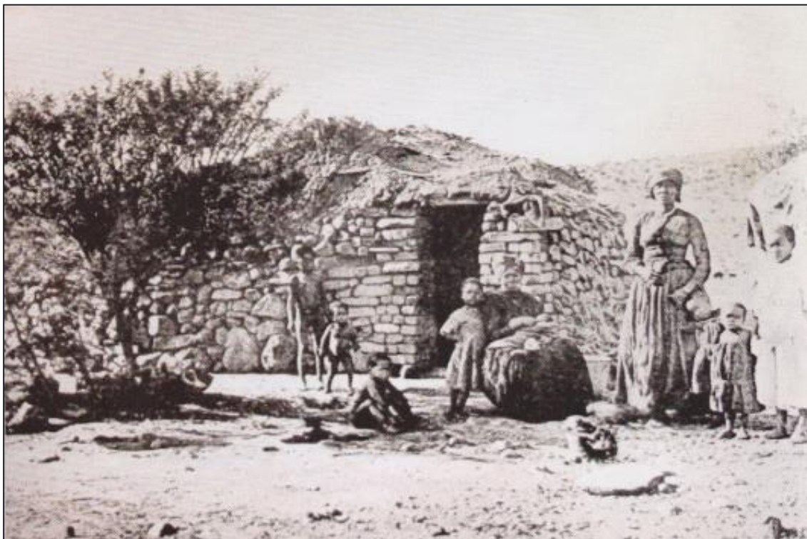
Figure 6-19 - A shepherd's hut photographed near Beaufort West in the early 20th century. Note the low, narrow doorway and informal roof structure. Source: Schoeman (2013:48)
