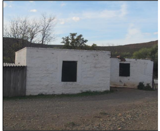
Figure 6-23 - Structure in the Leeukloof Farm complex at Waypoint 1850
