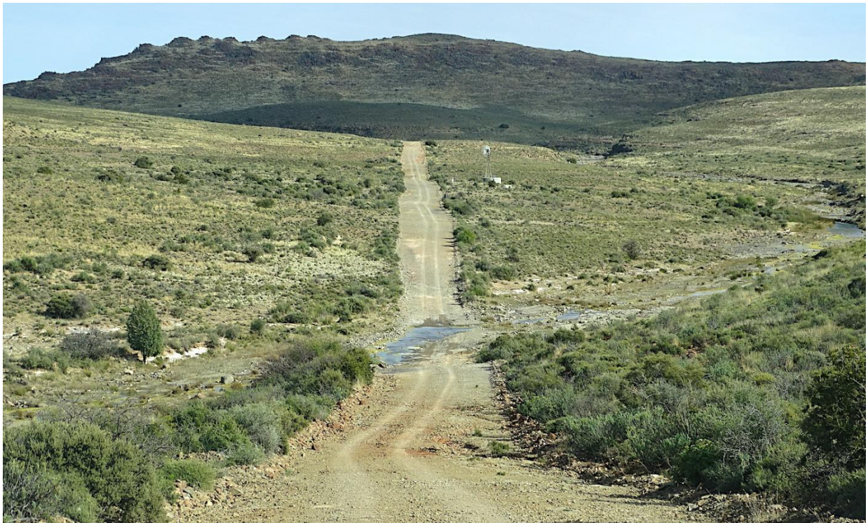
Figure 6-36 - Existing access road between Leeukloof and Boiskraal
