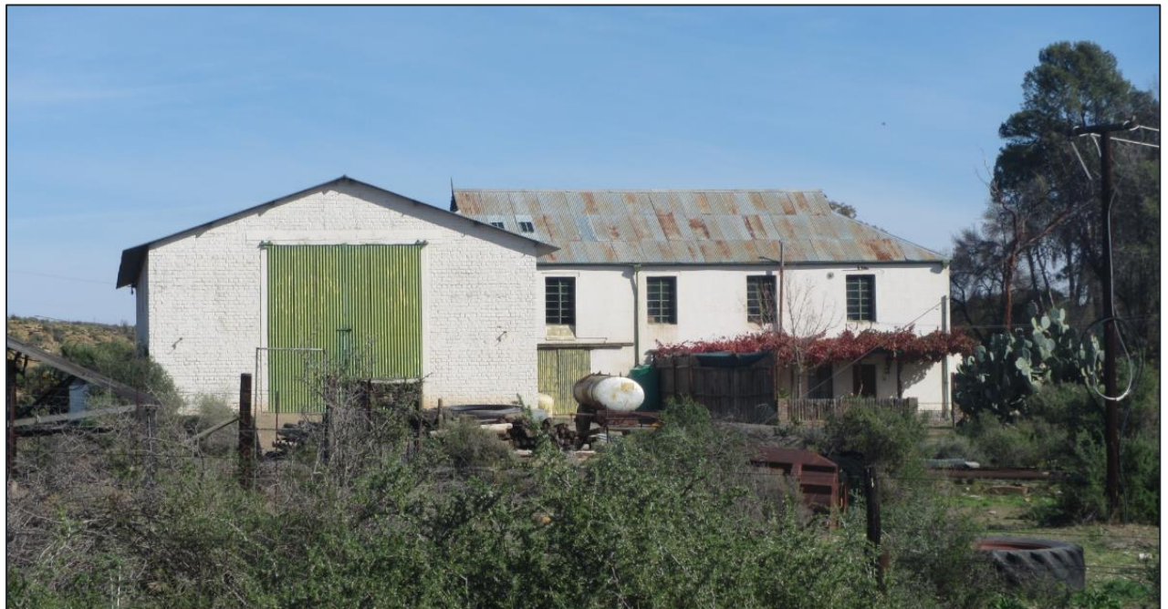
Figure 6-25 - A structure built of stone, sun-dried mud bricks and fired clay bricks at Waypoint 1993
