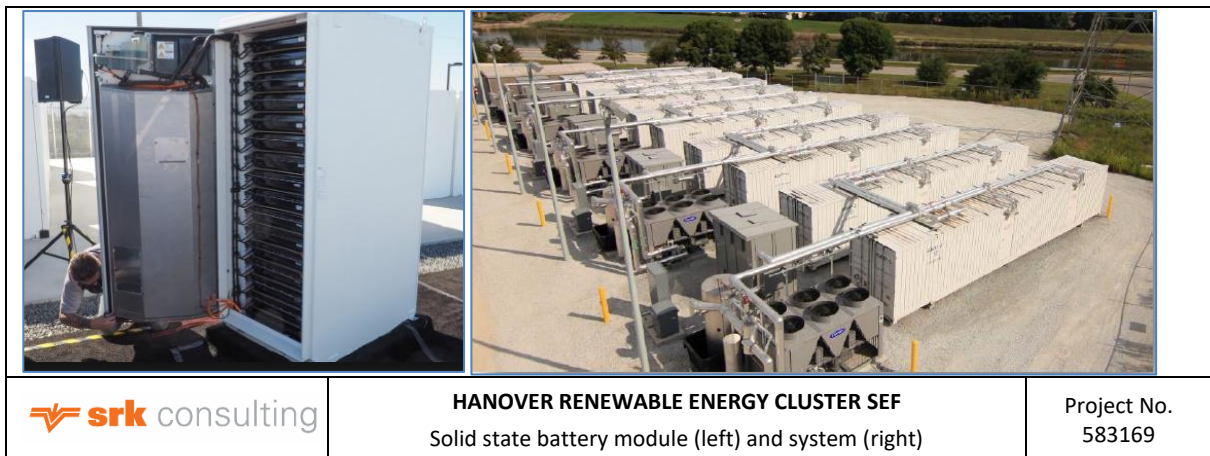
Figure 3-19: Solid state battery module (left) and system (right)
