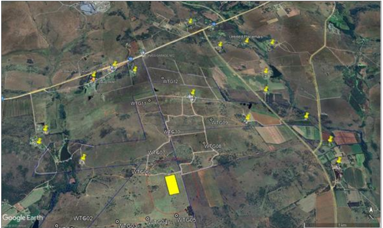
Figure 6-33 - Location of homesteads in the vicinity of the site (yellow place marks)
