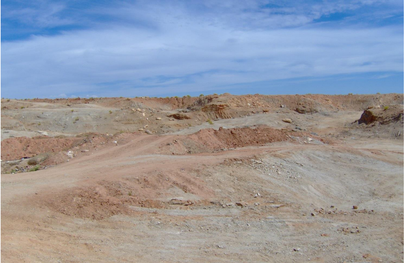
Photo 3: Floor of excavation to be kept level
