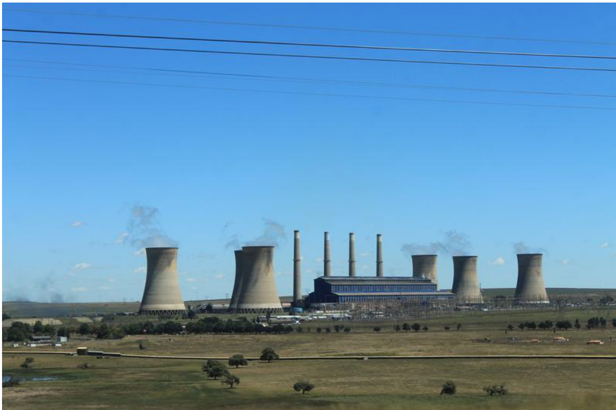
Figure 7-33: Camden Power Station
