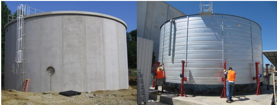
Figure 6-11: Typical water reservoir (left - concrete, right - steel)
