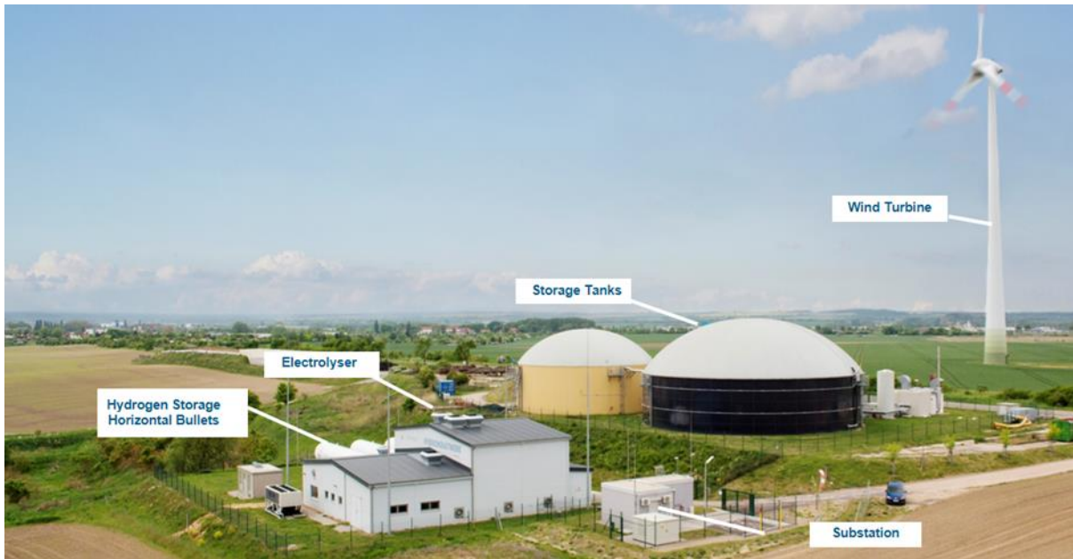
Figure 6-3: Enertrag Germany's Hybridkraftwerk
