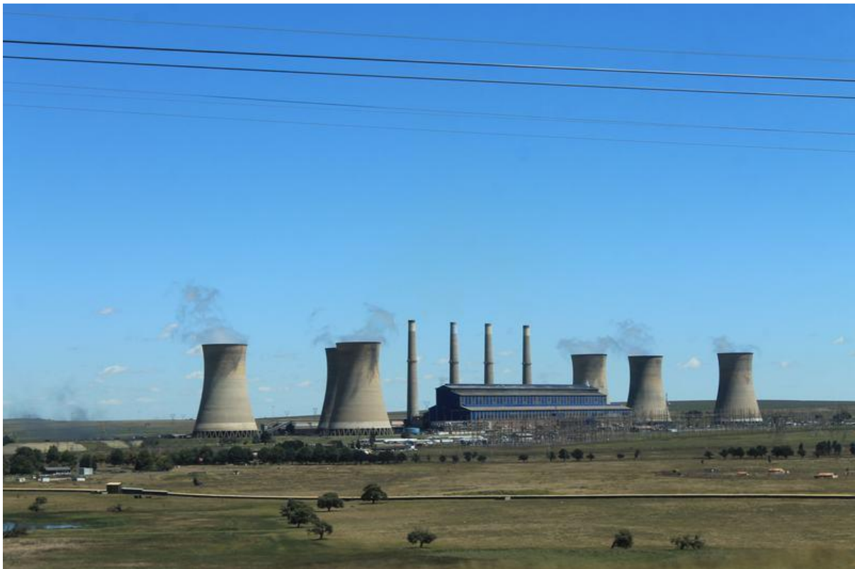
Figure 7.52: Camden Power Station
