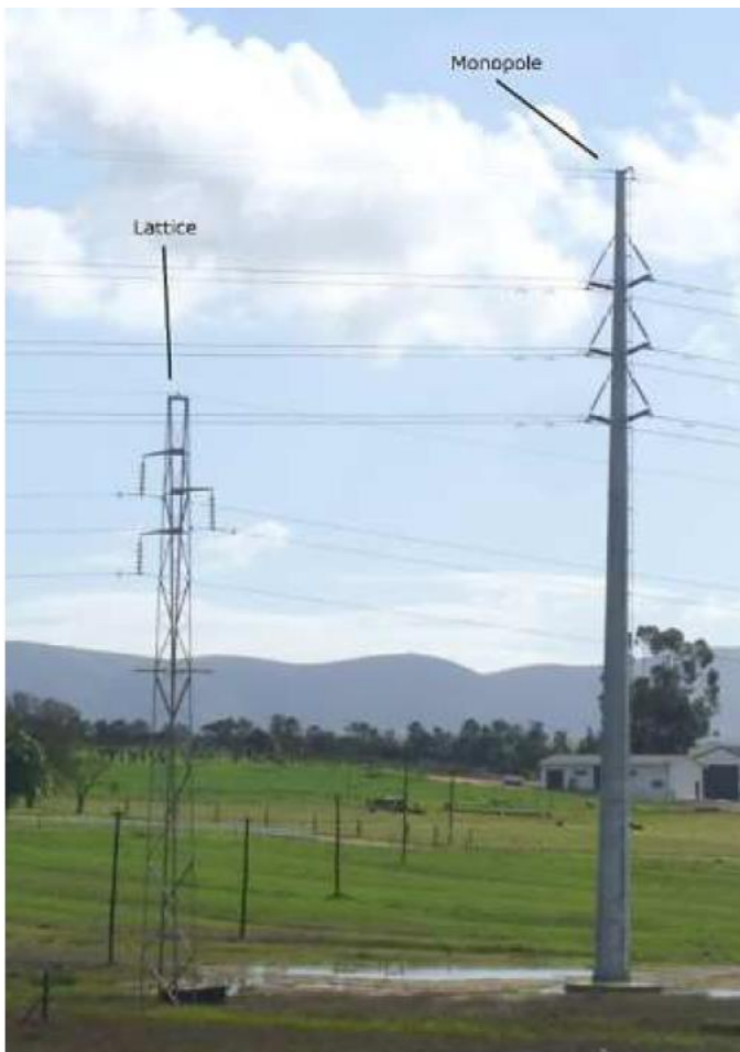
Figure 4-4: Conventional lattice powerline tower compared with a steel monopole structure
