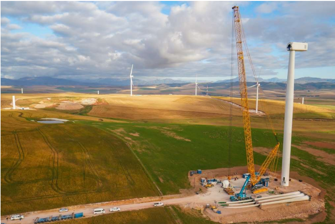
Figure 4-5: Construction of the Turbine – Lifting Equipment (i.e., Crane) (Source: BioTherm Energy, 2016)
