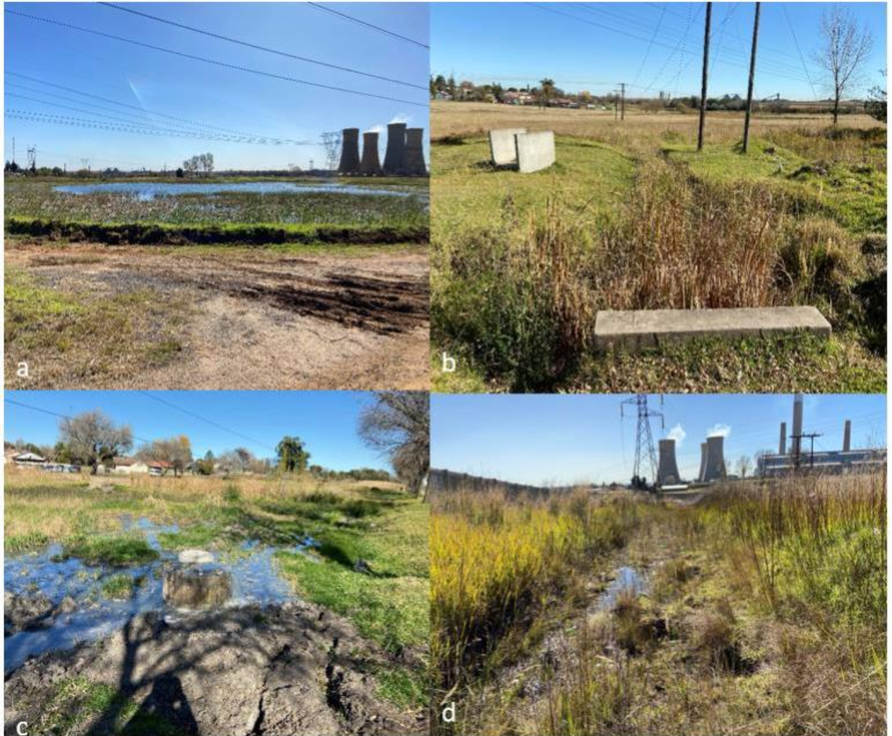
Figure 7-65 - Impacts: a) pooling of water at dam; b) trenches and berms in wetland; c) effluent discharge into the wetland from a leaking pipe; d) impoundment of water at roads in wetland
