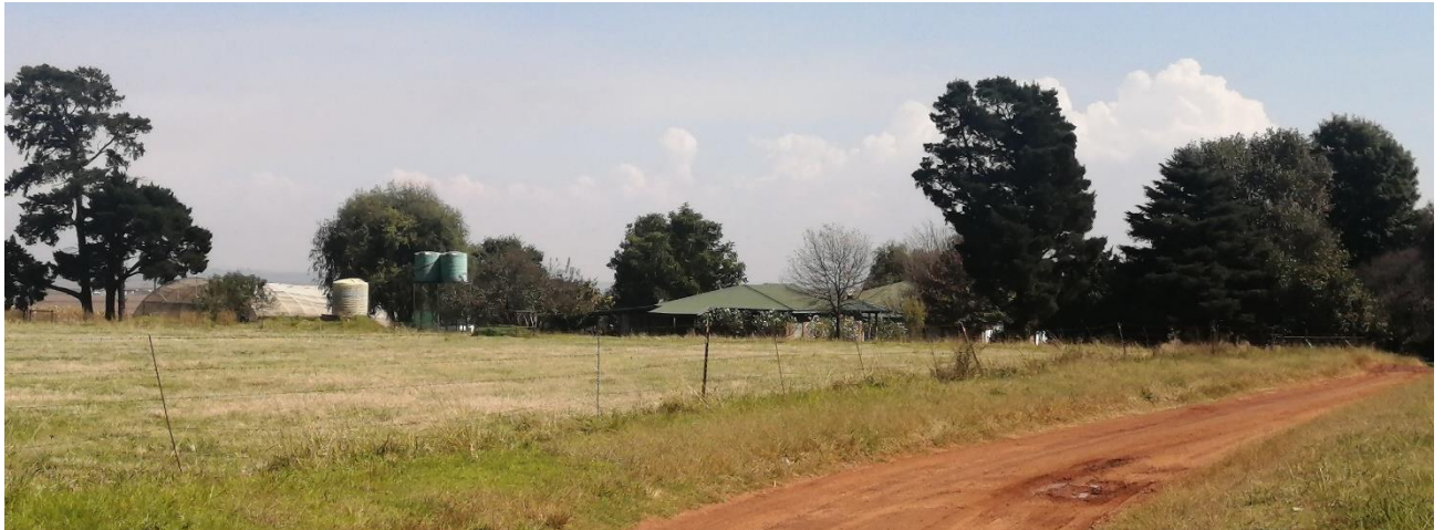
Figure 7-77: Example of a typical homestead located within the study area (LOGIS, 2023)
