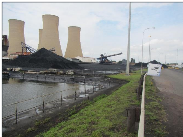
Figure 7-35 - The completely transformed coal deposit area at Komati Power Station
