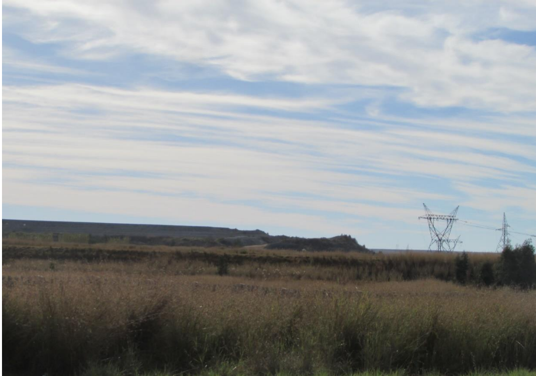
Figure 7-87: A view of the area with the Ash Discard Dump visible (APAC, 2023)
