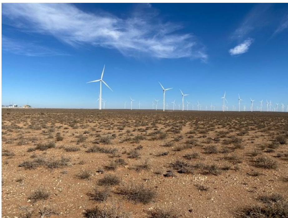
Figure 6-8: A view of the typical landscape where the grid alignment is located with the Khobab WEF substation far left on the horizon
