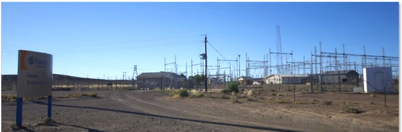
Figure 4-7: The Helios MTS east of the proposed Kokerboom WEF developments
