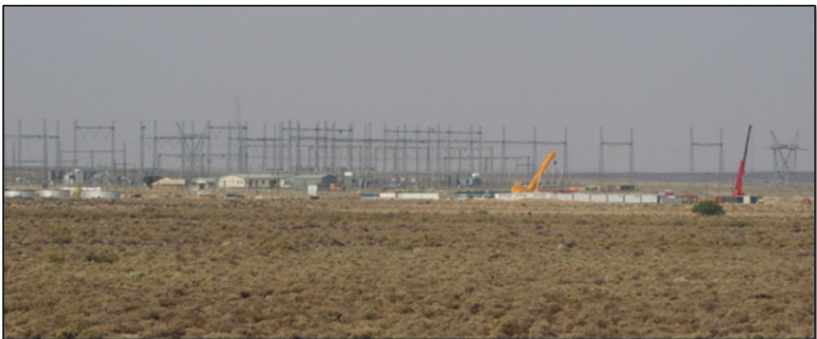
Figure 6-33: Photograph of the Eskom Helios substation.
