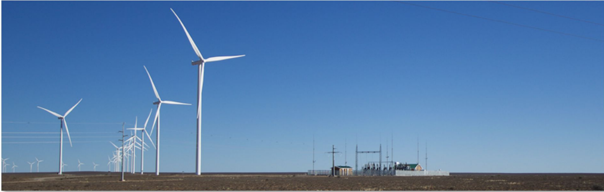
Figure 4-3: the existing Khobab WEF and substation in the foreground. Note the 132kV OHL situated “between” the turbines. Lat -30.436381°; Long 19.557894°; Direction W.
