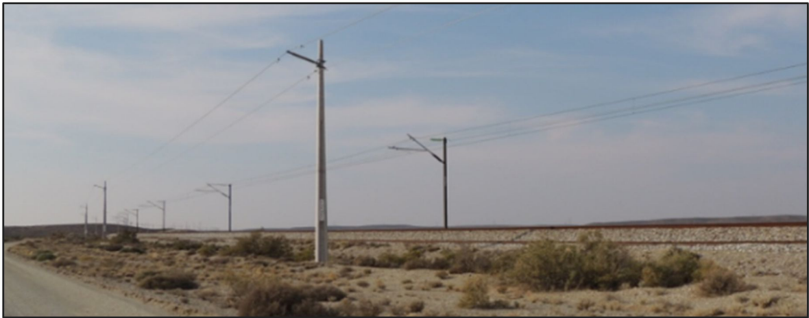
Figure 6-32: Photograph of the Shishen – Saldanha railway line.
