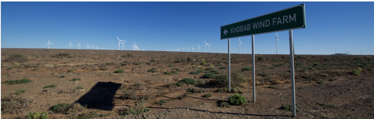
Figure 4-2: The existing Khobab WEF in the background. Lat -30.441436°; Long 19.557474°. Direction W.
