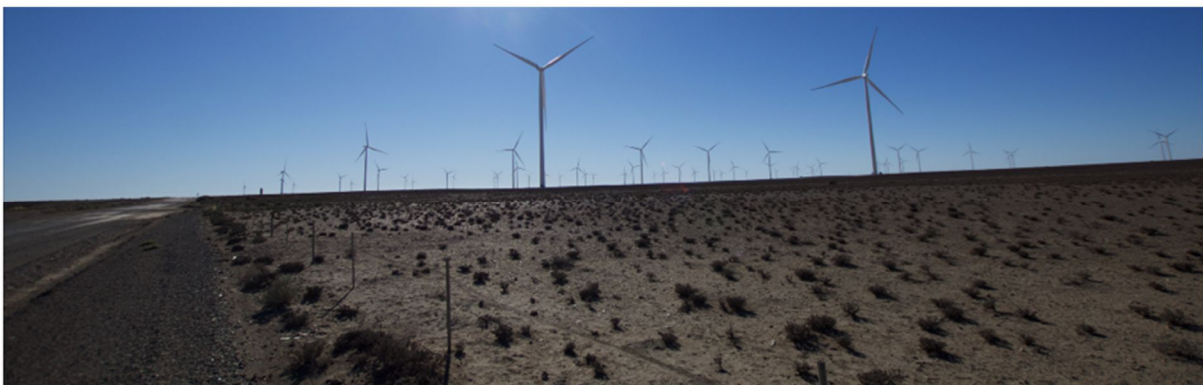
Figure 4-4: The Loeriesfontein WEF on the right. Lat -30.420416°; Long 19.561832°; Direction NE.
