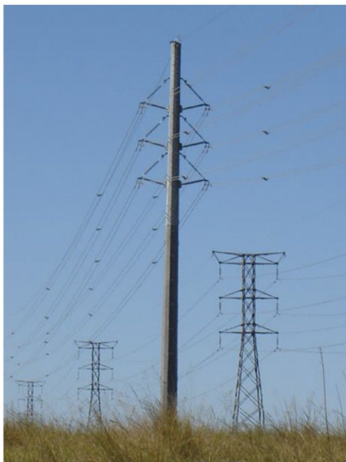
Figure 4-10: Example of a Self-supporting Monopole (foreground) and Lattice Structure (background)
