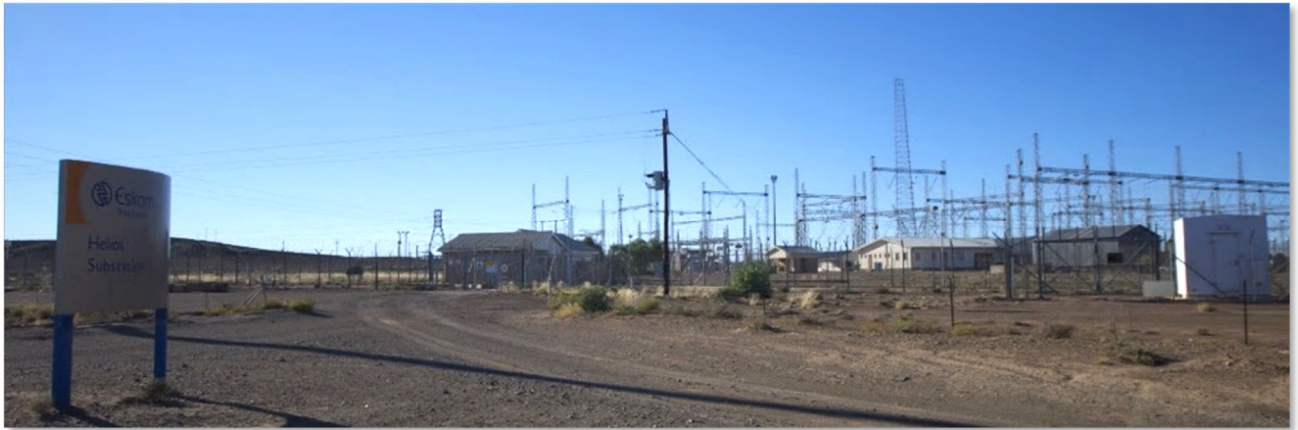
Figure 4-8: The Helios MTS east of the proposed Kokerboom WEF developments
