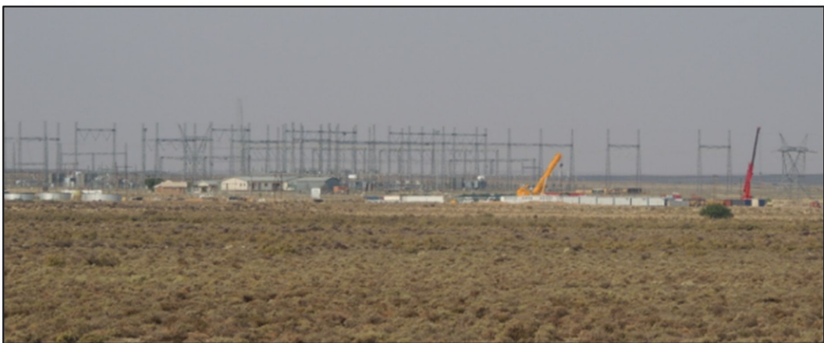
Figure 6-34: Photograph of the Eskom Helios substation.
