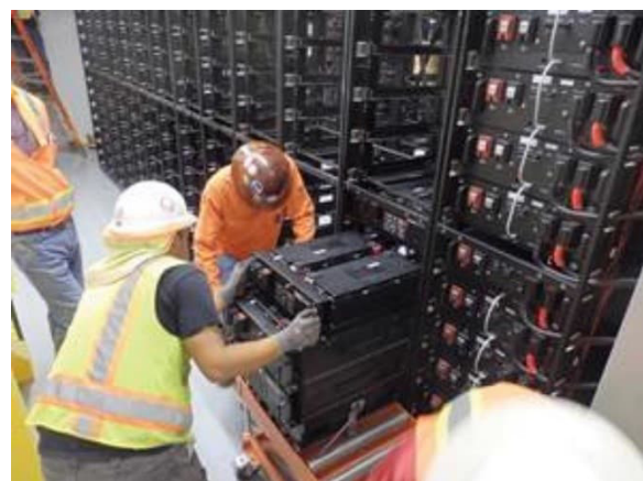
Figure 3-8 Typical Storage of Solid-State Battery Modules (within battery stacks)
