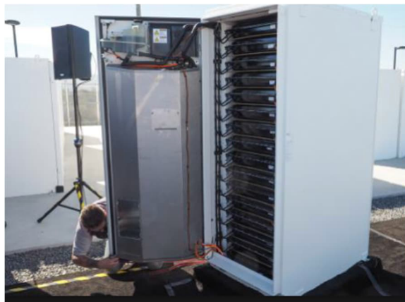
Figure 3-8 Typical Storage of Solid-State Battery Modules (within battery stacks)
