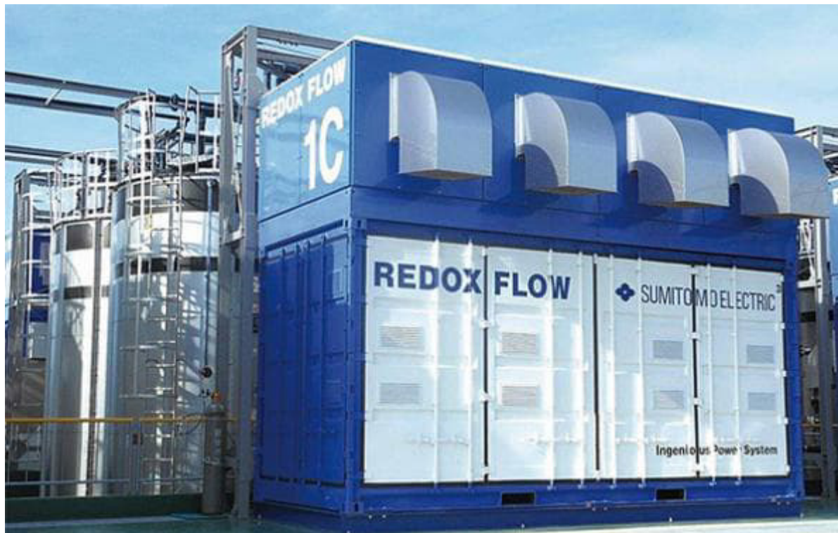
Figure 3-11 Standard BESS Design – VRF Flow Battery
