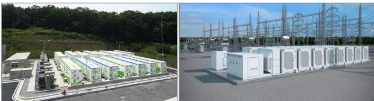
Figure 4: Typical configuration of Lithium-Ion BESS installed inside containers and blocks (EGP, 2022)
