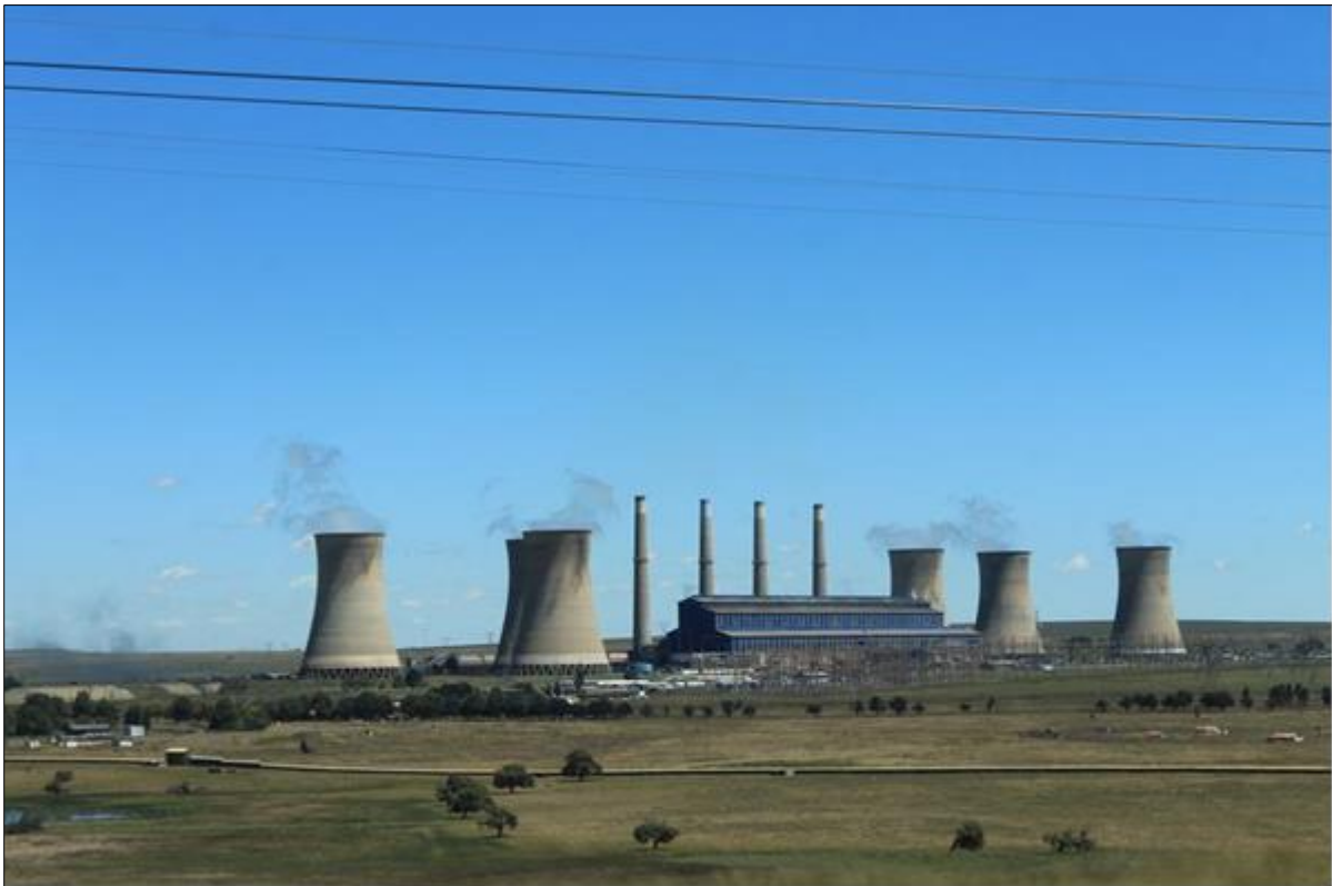
Figure 6-45: Camden Power Station
