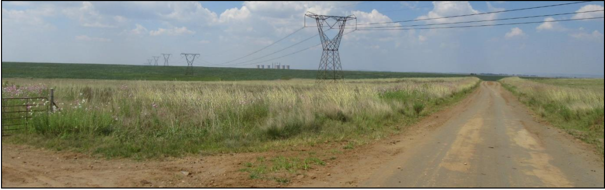
Figure 6-55: 400 kV line crossing the De Emigratie Road on Uitkomst
