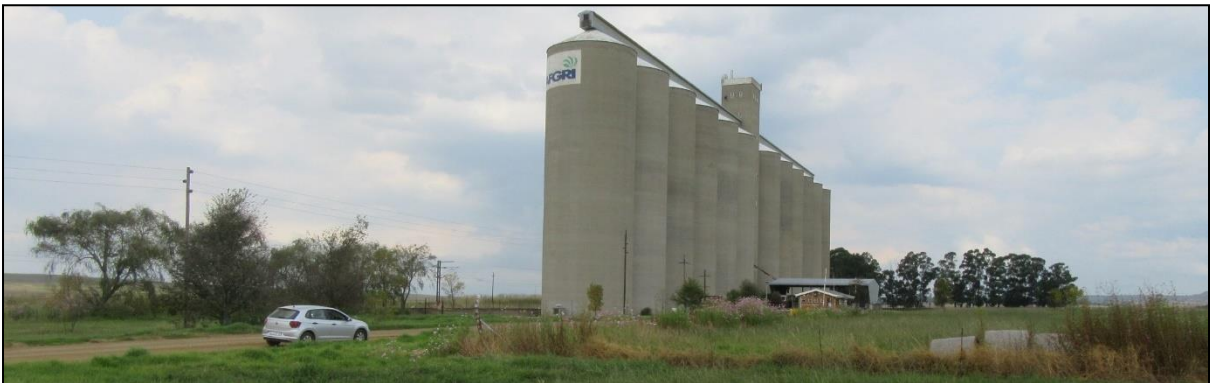
Figure 6-48: Overvaal silo located adjacent to the Richards Bay railway line
