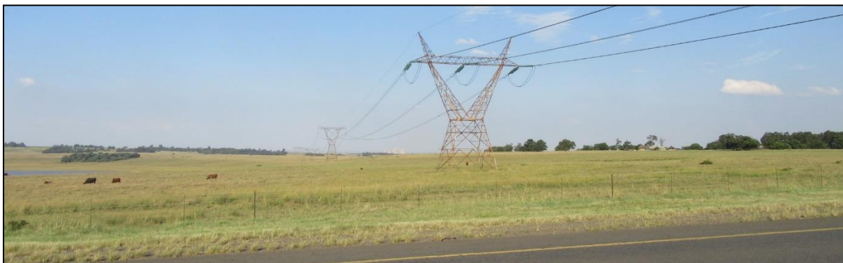
Figure 6-54: 400 kV line crossing the N11 approximately 6 km south of Ermelo
