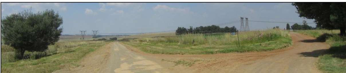
Figure 6-43: Two 400 kV lines traversing De Emigratie Road
