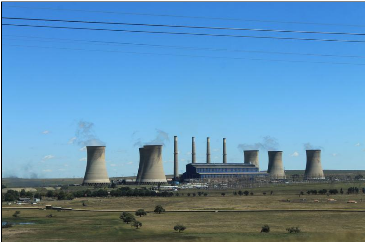
Figure 6-34: Camden Power Station
