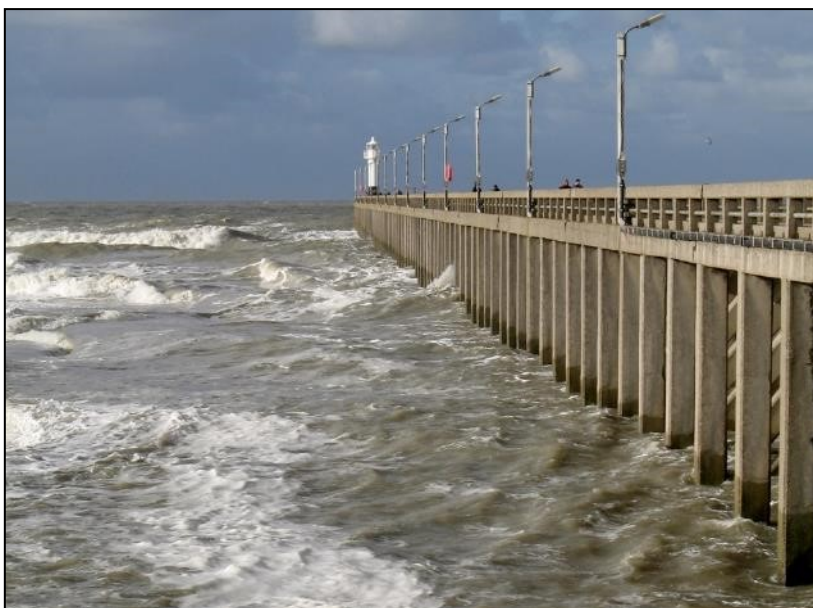
Plate 2.4: Example of intake jetty.
