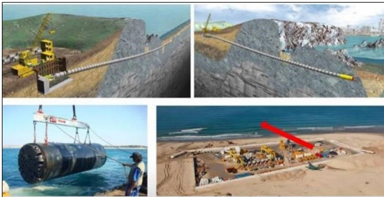
Plate 2.6: Illustration of the on-land launch shaft and jacking process during the tunnelling process (WSP, 2020).
