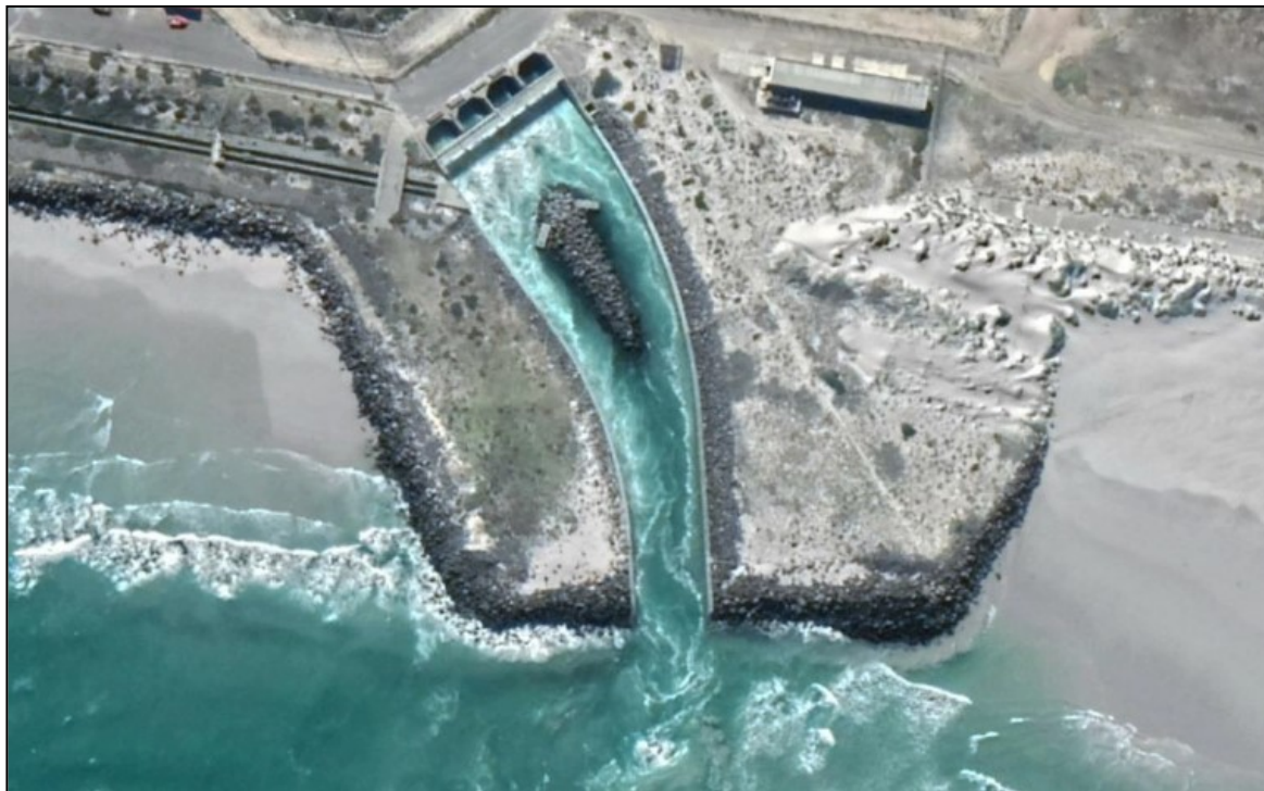
Plate 2.5: Typical outfall raceway found at the Koeberg Nuclear Power Plant (WSP, 2020).
